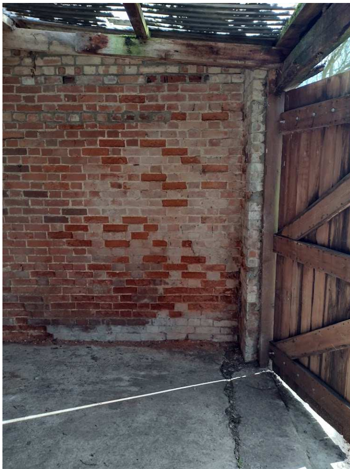
PHOTOGRAPH B – SECTION 2
