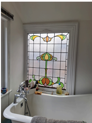
Fig. 12. Existing window in party wall between No 54 and 56. To remain in place.
