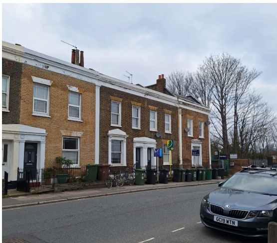
Fig. 2. Existing front facade
