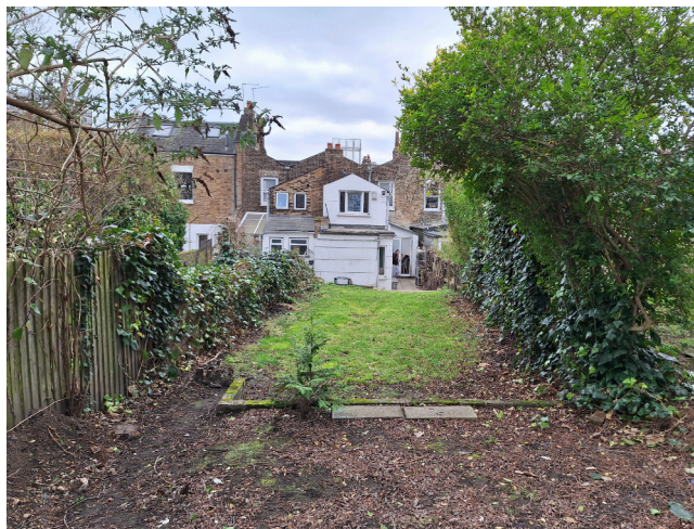
Fig. 3. Existing rear facade seen from garden end
