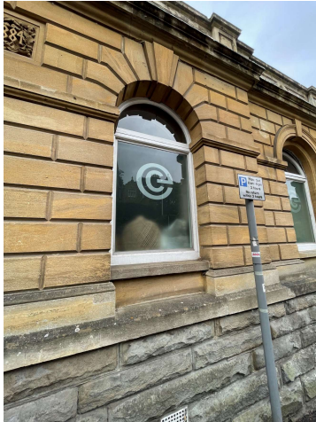
Existing windows to Banking Hall. New windows to be installed and cill lowered to original size.
