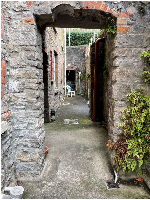
View of rear passage
