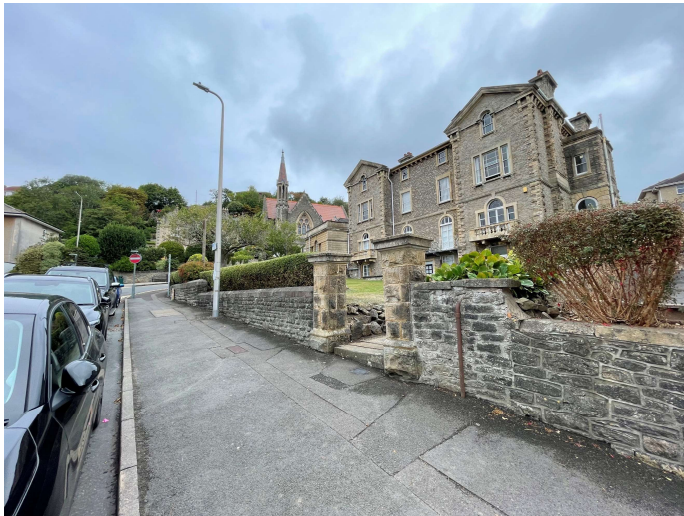
View of existing pedestrian access
