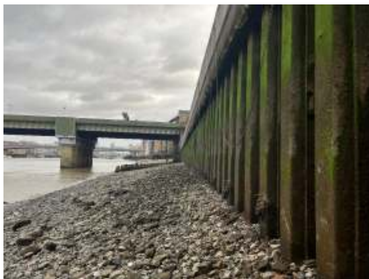
Photograph 3.1 – General view along the sheet piled wall
