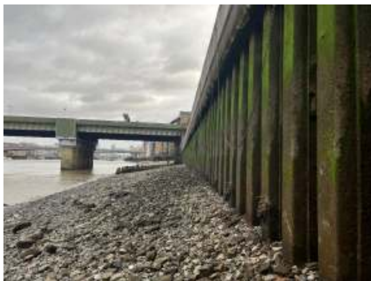
Photograph 3.1 – General view along the sheet piled wall
