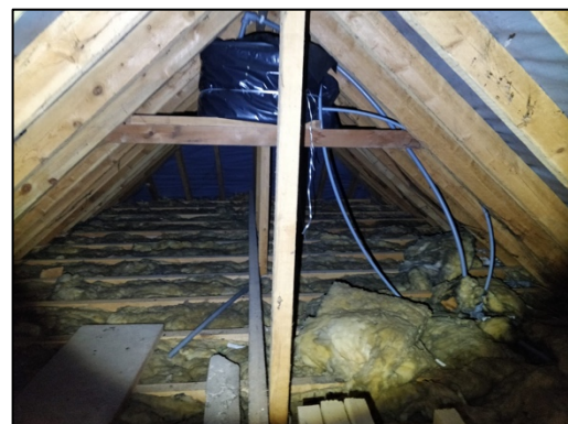
Figure 4 – roof void inside the southern extension
