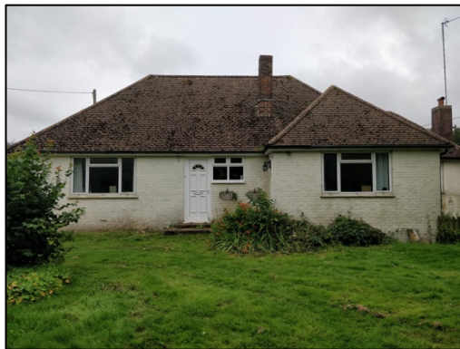
Figure 1 – northern elevation and extension
