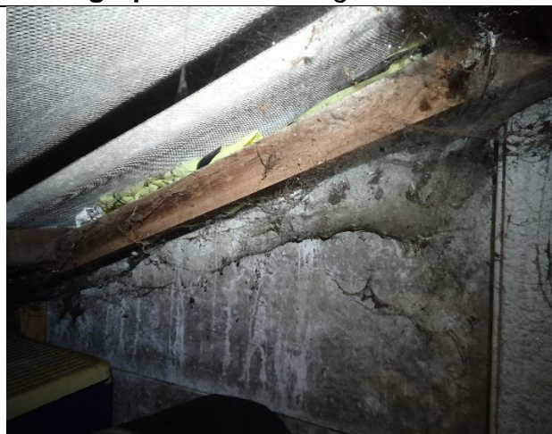
Photograph 8: Highly cobwebbed roof void with sealed verges
