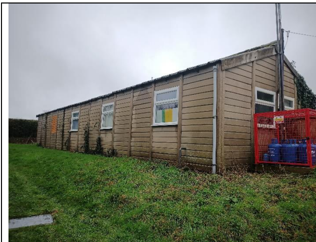
Photograph 5: North and east elevations
