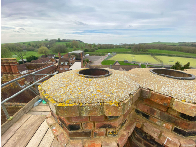
Flaunching and liner
