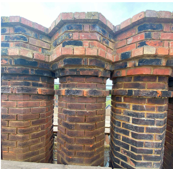
Flue stacks south central chimney A
