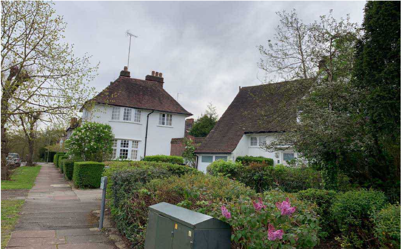
View to number 46 Temple Fortune Hill showing the end elevation bay window and number 44 forming the end house to Crickmer Circus to the right.
