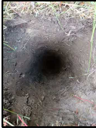
Hand-dug starter pit: 0.00-1.00m
