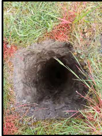
Hand-dug starter pit: 0.00-1.00m
