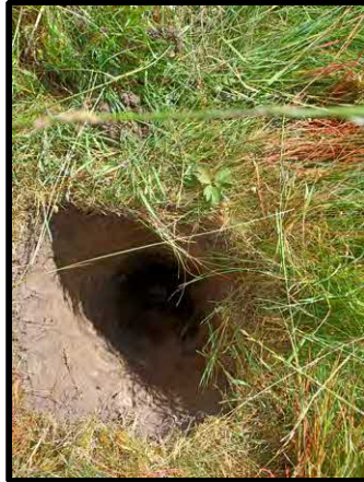
Hand-dug starter pit: 0.00-1.00m
