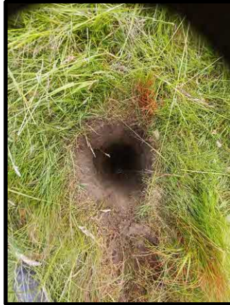
Hand-dug starter pit : 0.00-1.00m
