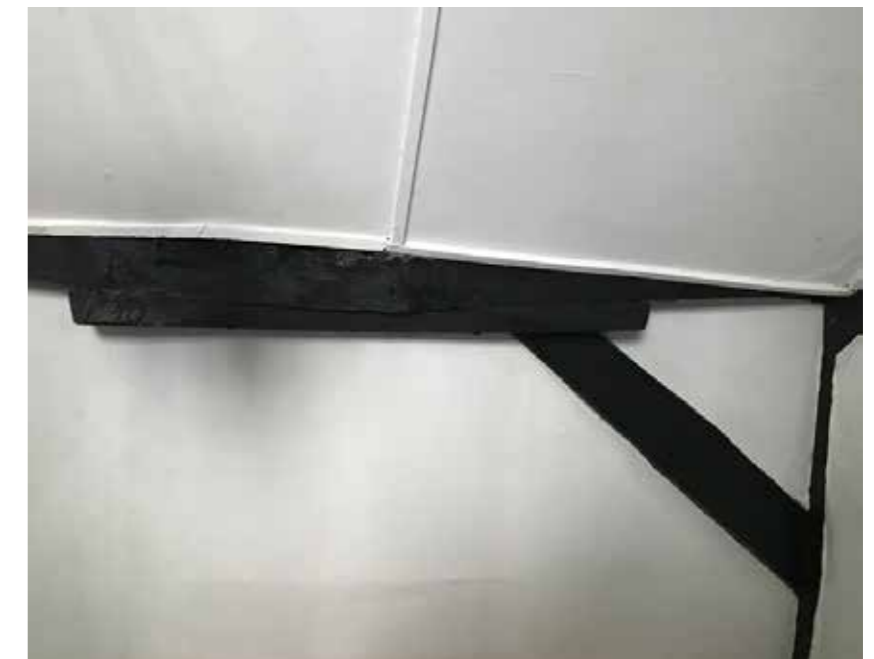
Above left + right: Rafters bay 4, showing redundant hip rafter
