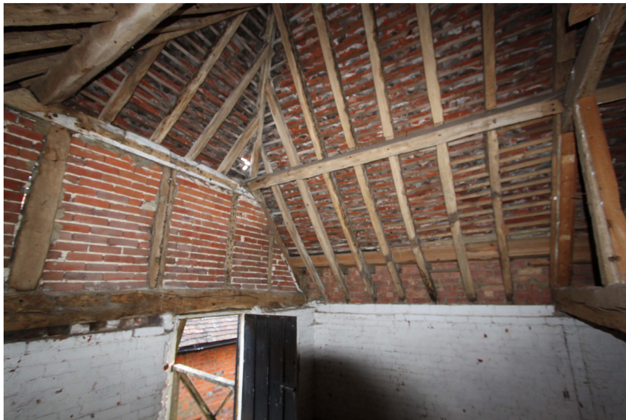
Renewed roof timbers
