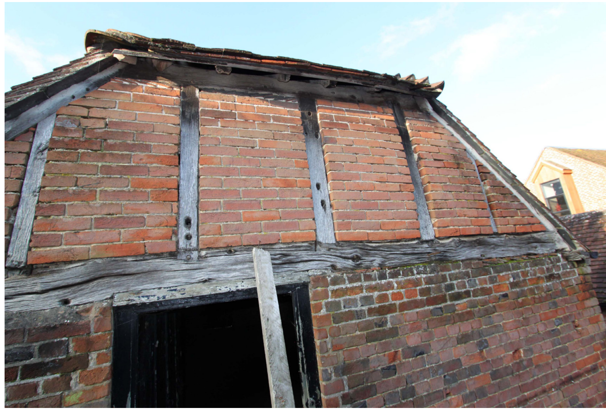
Existing building rear first floor
