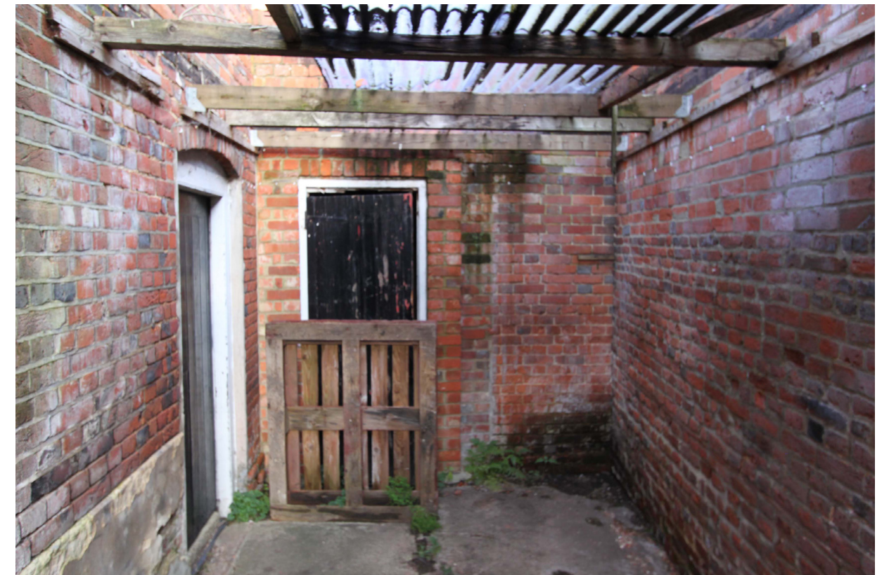
Existing outbuilding (WC block)
