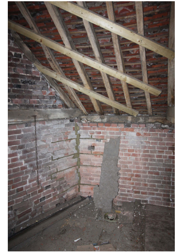
Replacement (not original) roof timbers
