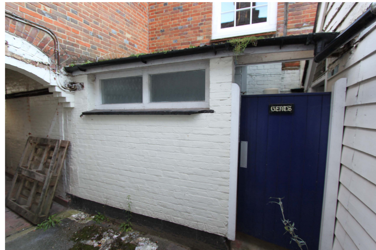
Existing outbuilding (WC block)
