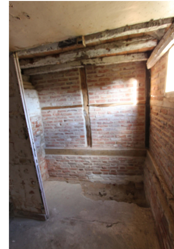
Recently repaired stock brick and Oak frame wall
