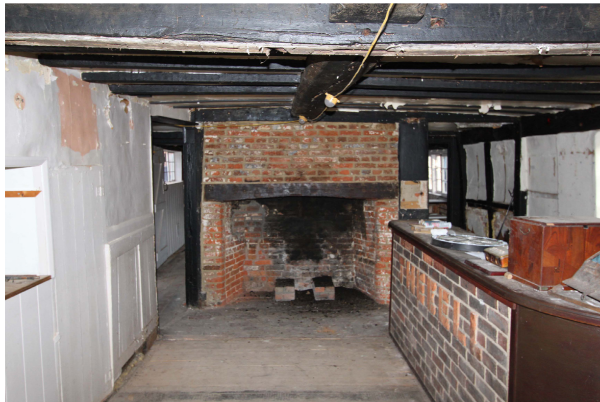
Existing buildings interior
