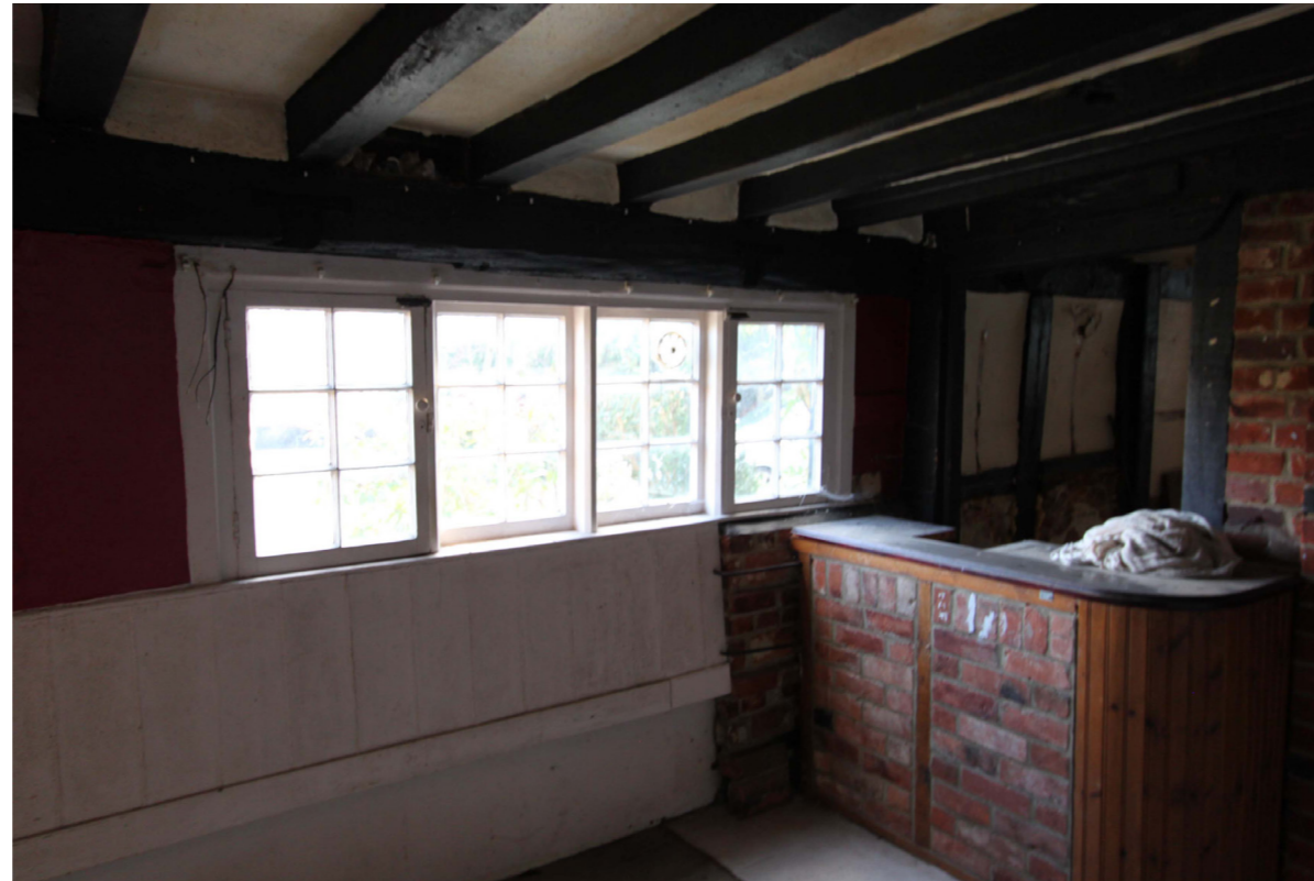
Existing building interior
