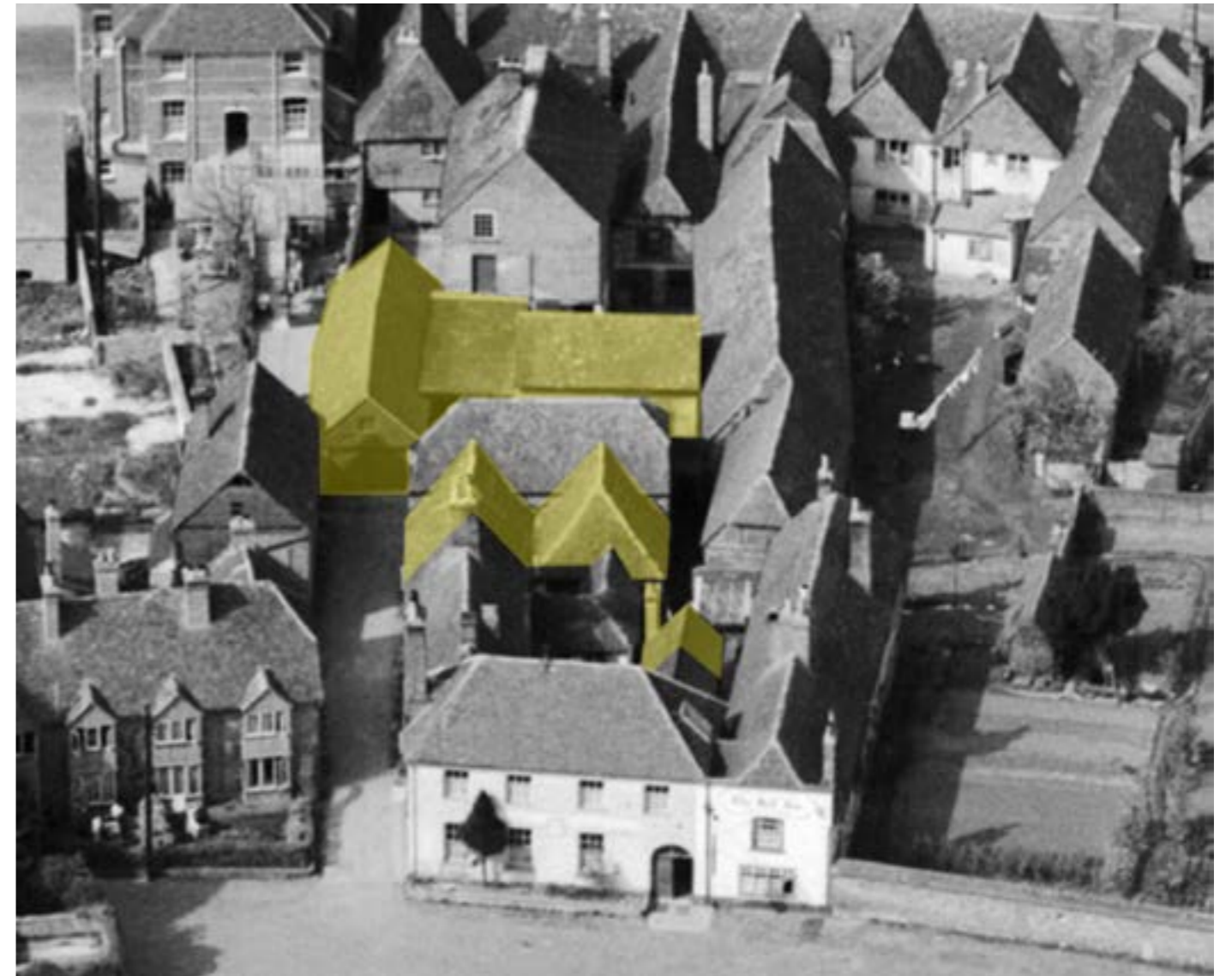
Detail from a photograph taken in 1949 of the former service yard, now known as Terry's Alley. Structures shaded yellow have since been demolished
