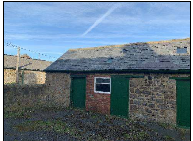
Photograph 4 Building Reference 2, south elevation.
