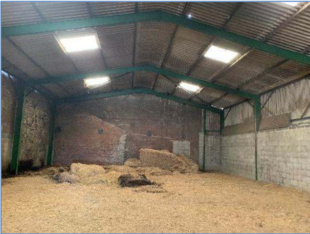
Photograph 13 Building Reference 7, internal.
