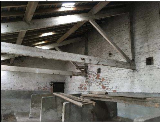
Photograph 19 Building Reference 9, internal.
