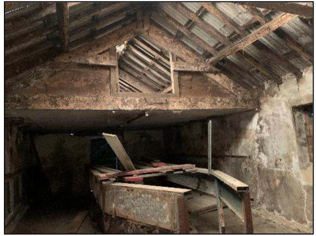
Photograph 10 Building Reference 5, internal showing loft.
