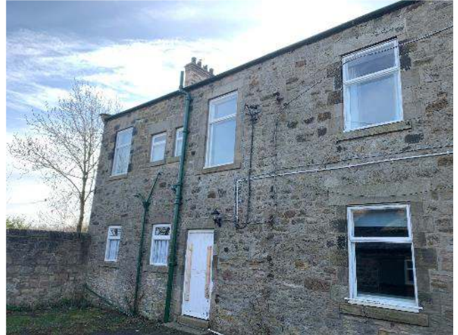
Photograph 2 Building reference 1, Farmhouse.
