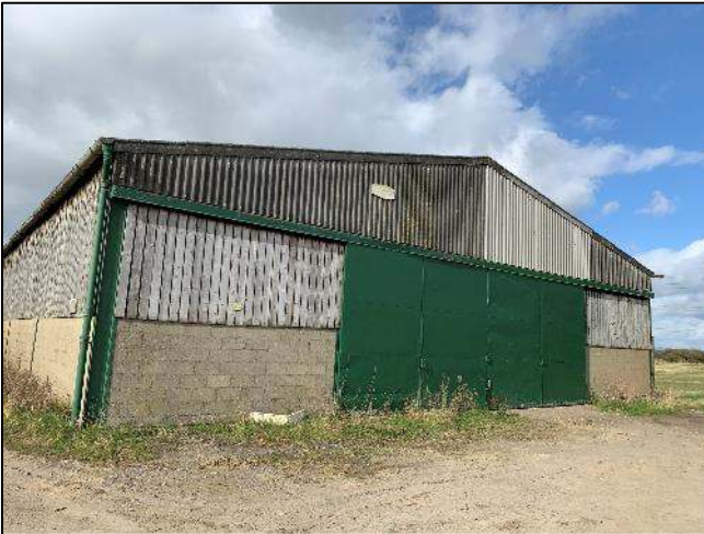
Photograph 21 Building Reference 11, external.
