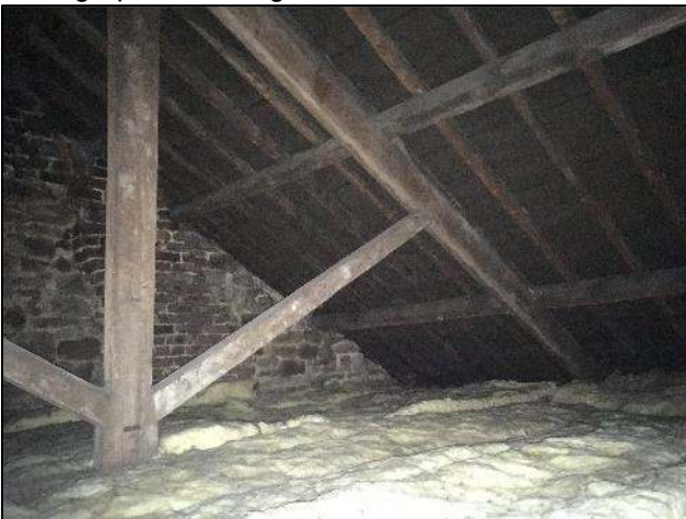
Photograph 3 Building Reference 1, inside loft void.
