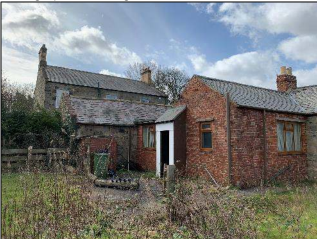
Photograph 5 Building Reference 2 & 3, showing gaps in the roof of 2.
