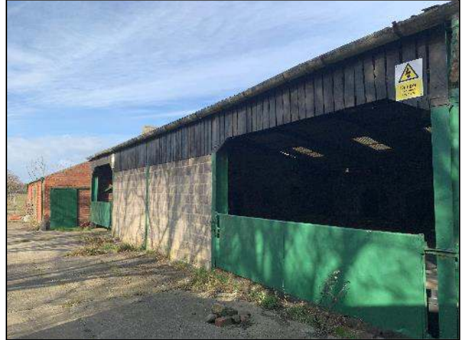
Photograph 18 Building Reference 9 & 10, external
