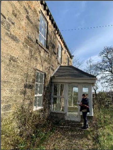
Photograph 1 Building reference 1, Farmhouse.
