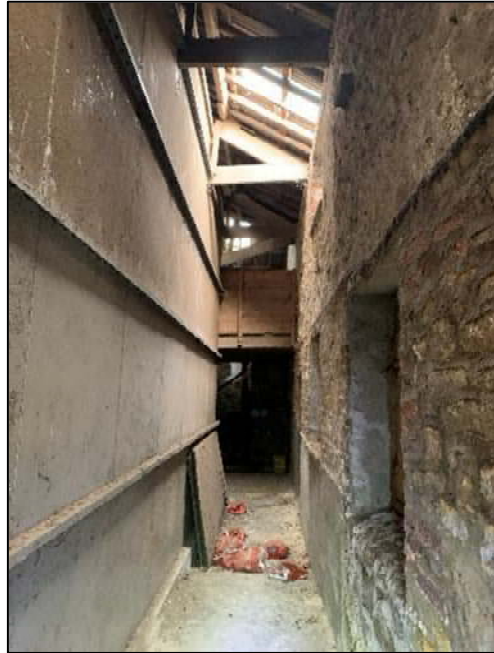
Photograph 14 Building Reference 8, internal.
