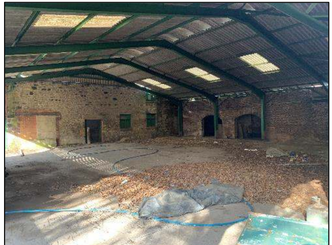
Photograph 20 Building Reference 10, internal.
