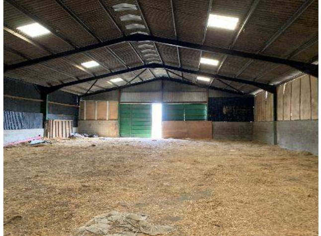
Photograph 22 Building Reference 11, external.
