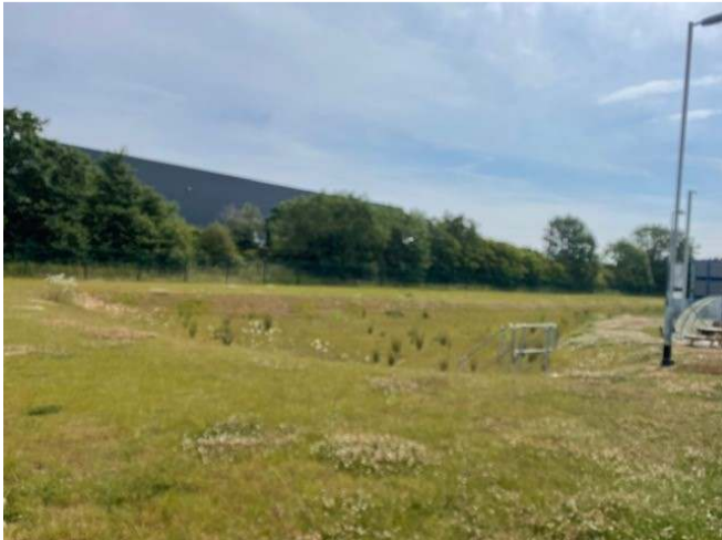
Photograph 6, Pond 6 – dry SuDS pond within Faltec.
