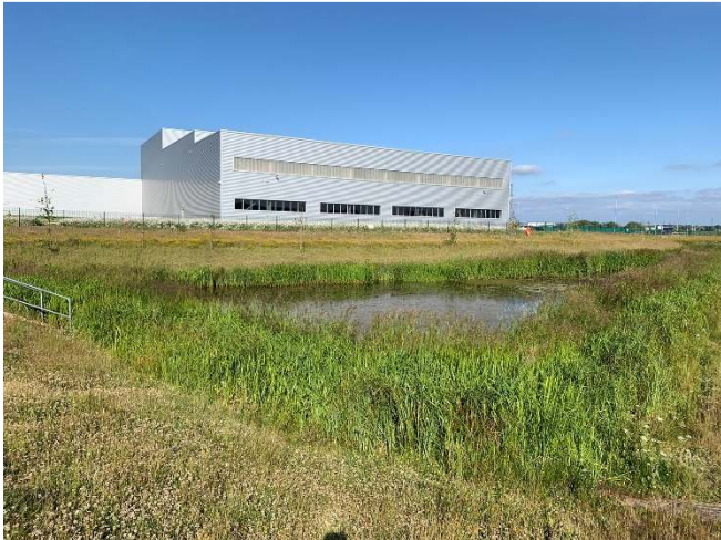
Photograph 10, Pond 10 middle SuDS Pond.
