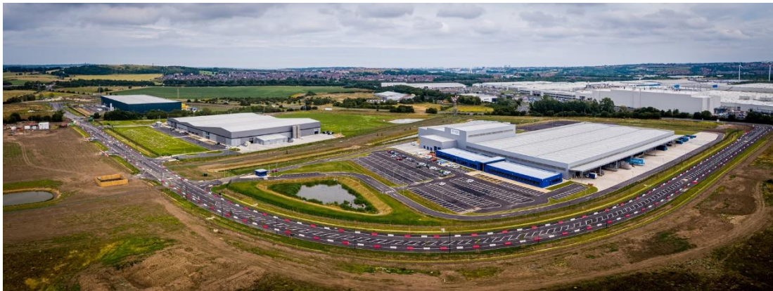
Figure 2.3 Photograph of the three industrial units looking eastwards
