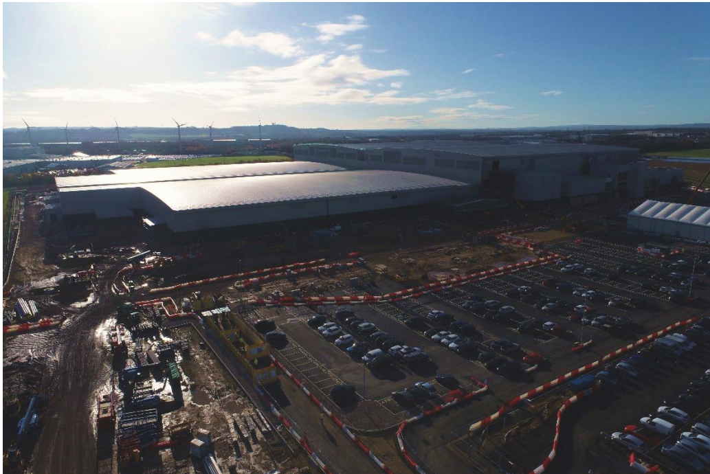
Figure 3.2 AESC Plant 2 under construction
