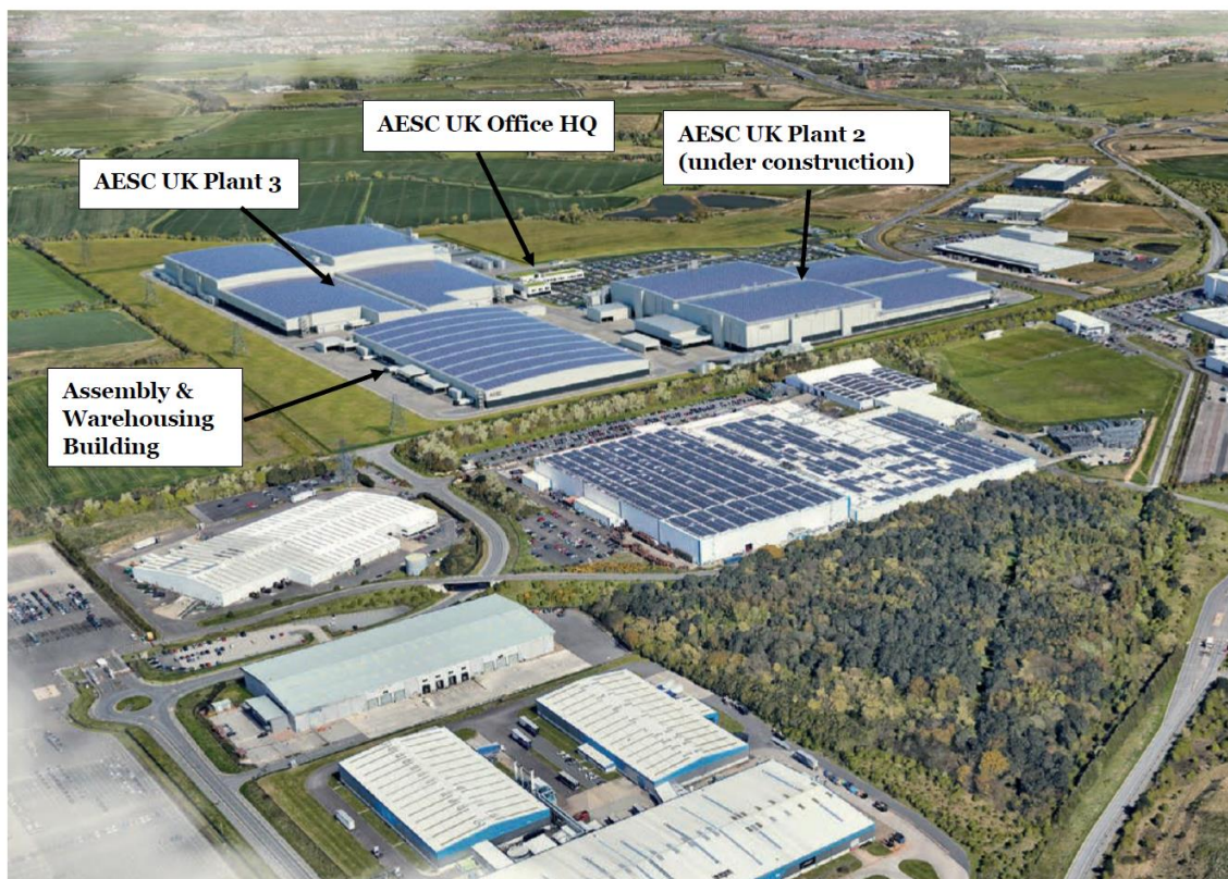
Figure 4.1: CGI of the proposed AESC Plant 3 development and AESC Plant 2 (under construction)
