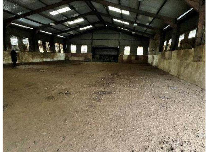
Photograph 2 Building reference 2, internal.
