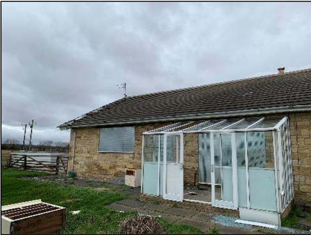
Photograph 7 Building Reference 5, farmhouse.
