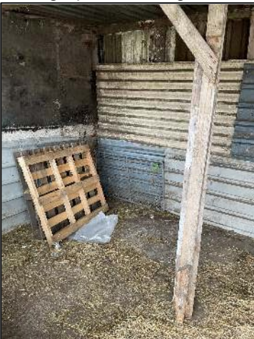
Photograph 5 Building Reference 3 internal where barn owl pellets were found.
