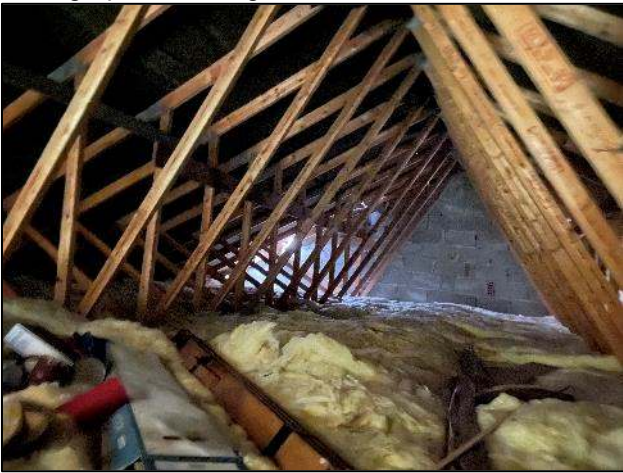
Photograph 9 Building Reference 5 loft void.
