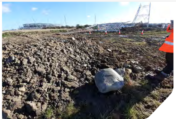
Photo 12: Pylon under construction, boulders from excavated soils in foreground.
