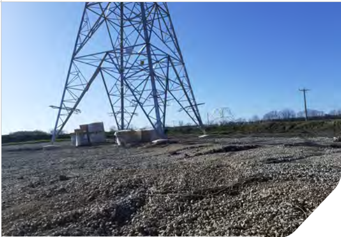
Photo 09: Newly constructed electricity pylon
