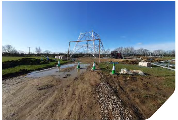
Photo 10: Electricity pylon under construction
