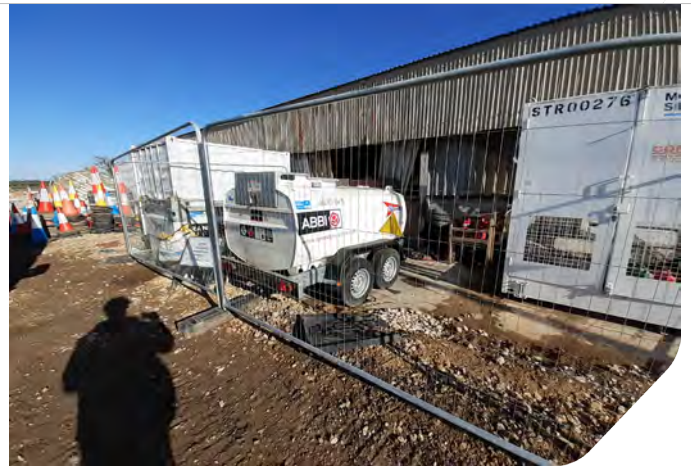
Photo 04: North Moor Farm fuel storage area
