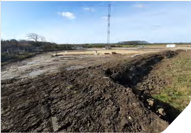
Photo 15: Temporary Pylon in power line realignment
