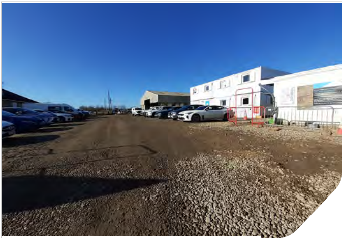
Photo 01: North Moor Farm, parking and offices
