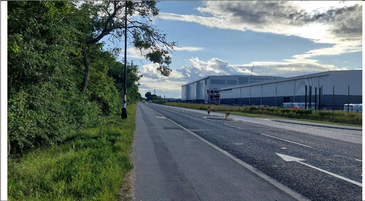
Location 21 junction with A1290/International Drive showing the AESC Plant 2 site
