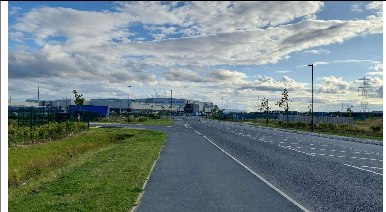
Existing lighting at location 20 International Drive
