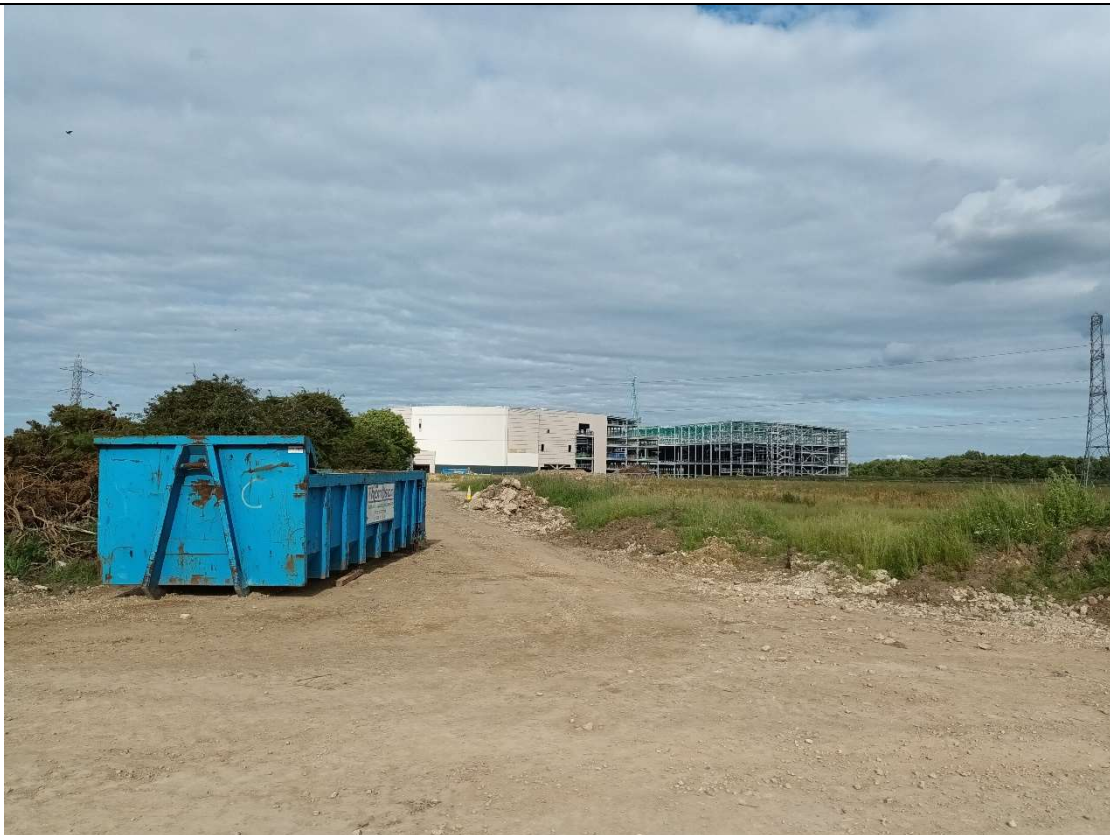
Location 2 from within the scheme extents towards AESC Plant 2.
