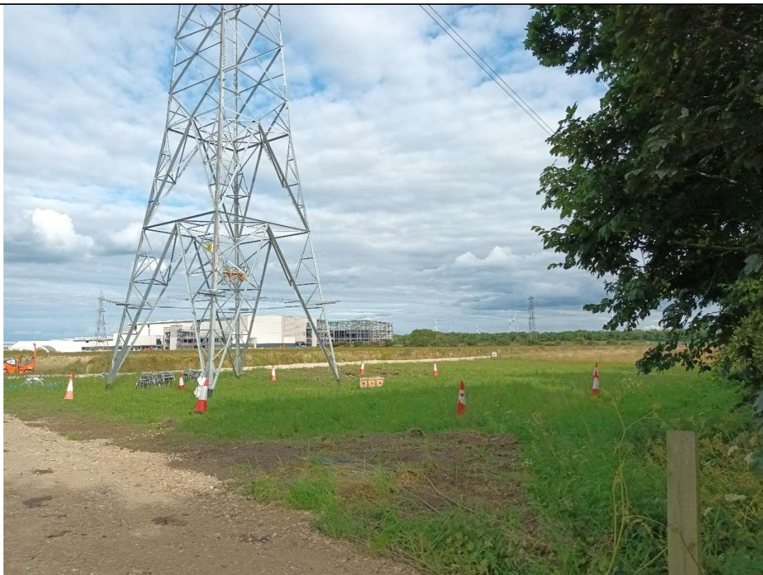
Location 7 from boundary line back into the Site towards AESC Plant 2.
