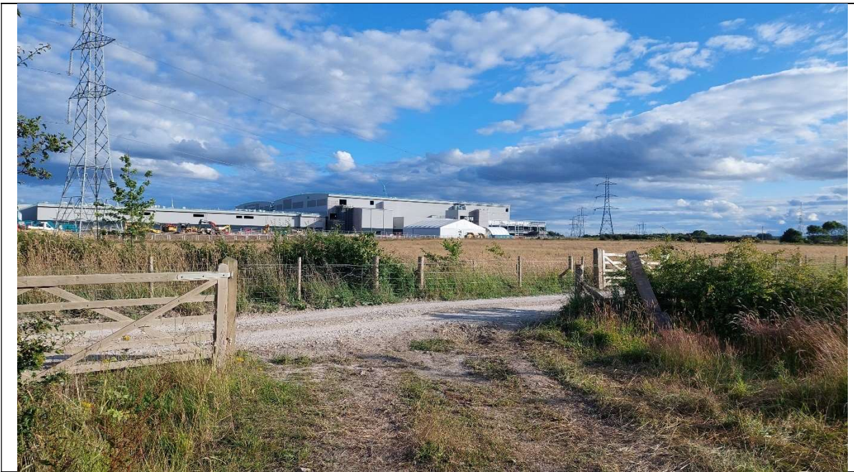
Location 19 across towards AESC Plant 2 site
