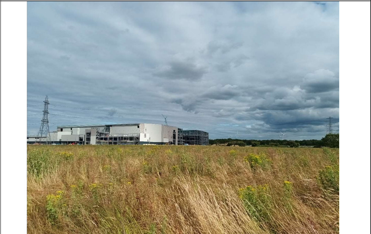
Location 1 from within the scheme extents towards AESC Plant 2.
