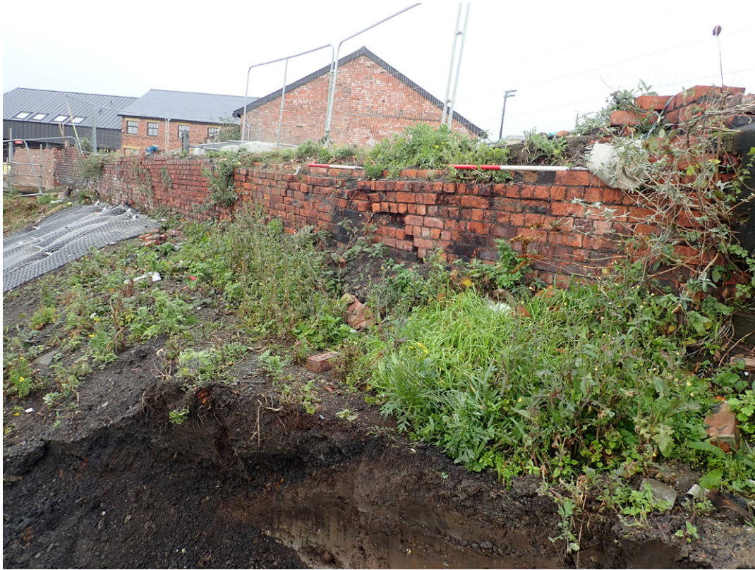
Fig. 3.33: South elevation of Grade 2 listed Wall 604, facing north-west
