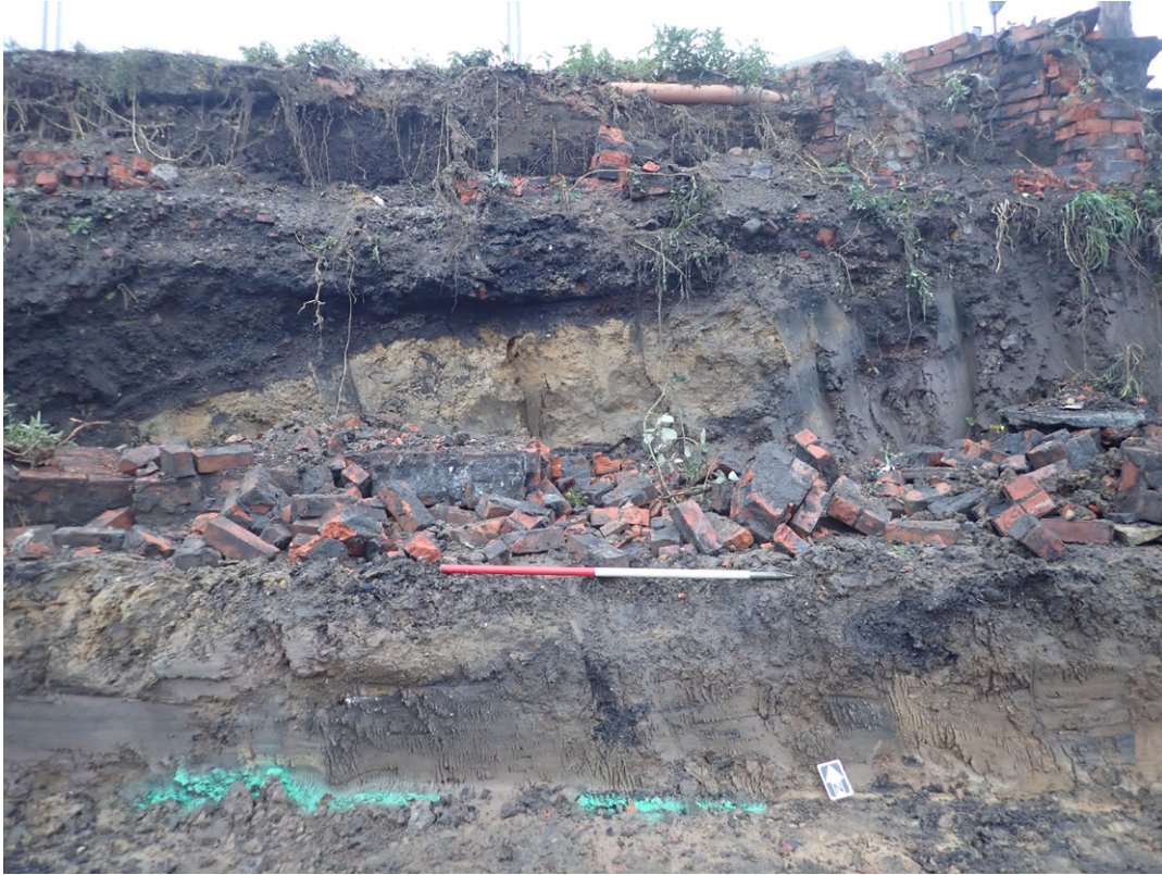
Fig. 3.35: South facing representative section in North Abutment, showing concrete Structure 605, and Made Grounds 602 and 603
