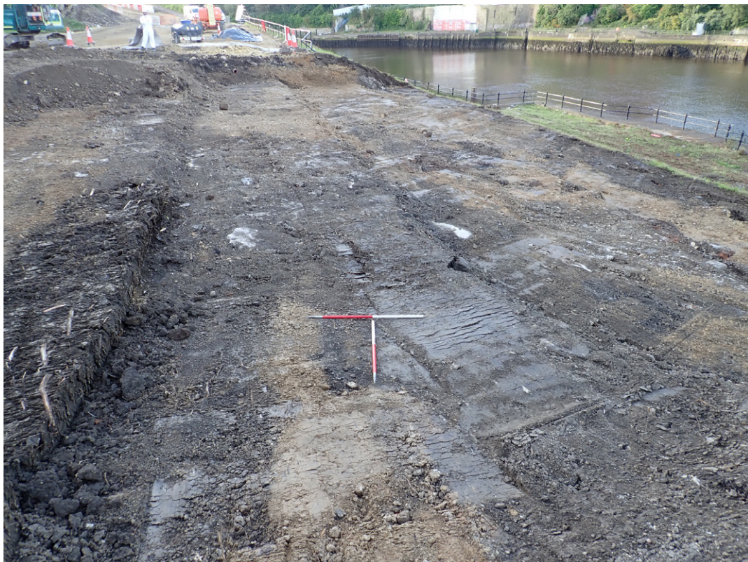
Fig. 3.4: Excavation to required depth in Area 1, facing south-east
