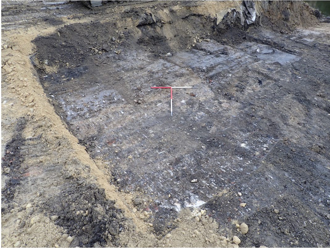
Fig. 3.5: Excavation to required depth in Area 1, facing south-east
