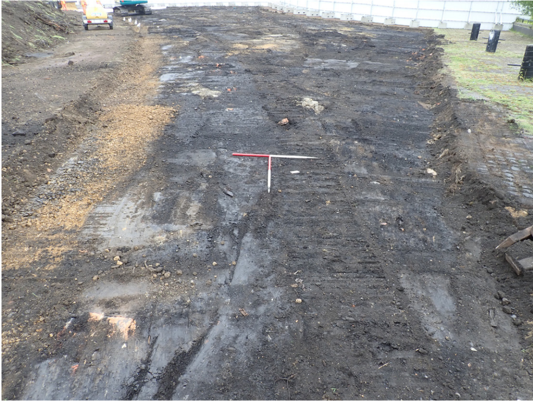
Fig. 3.23: Excavation to required depth in Area 3, facing west
