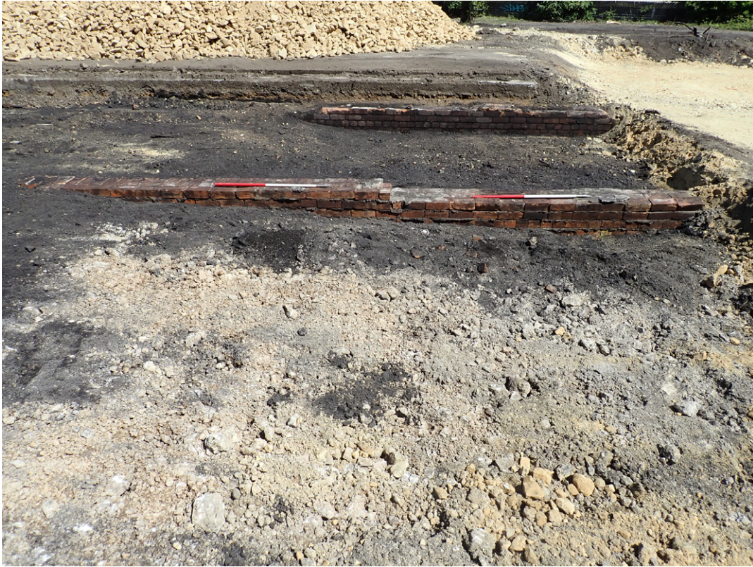
Fig. 3.21: South elevation of Wall 207
