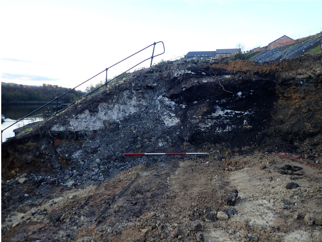
Fig. 3.25: East facing representative section in North Pier, showing Made Ground 502 and modern staircase with foundation layer of chalk
