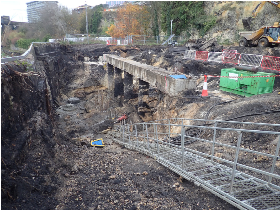
Fig. 3.40: Excavation to required depth in South Pier pit, facing south-east
