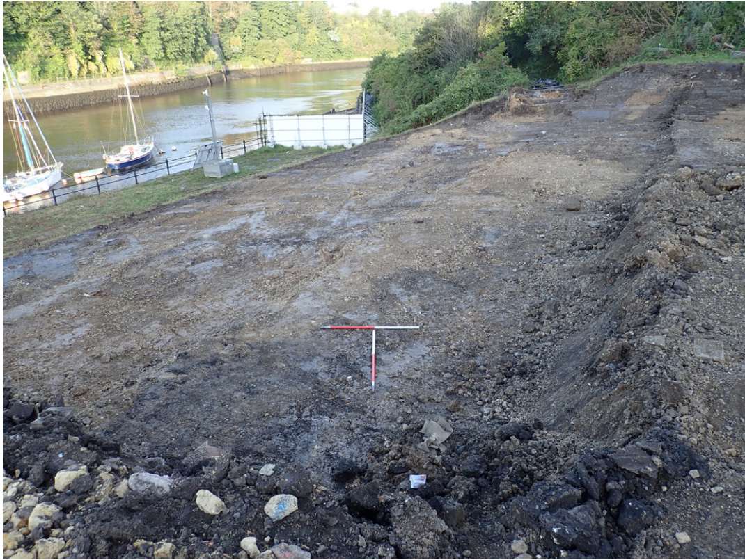
Fig. 3.3: Excavation to required depth in Area 1, facing south-west
