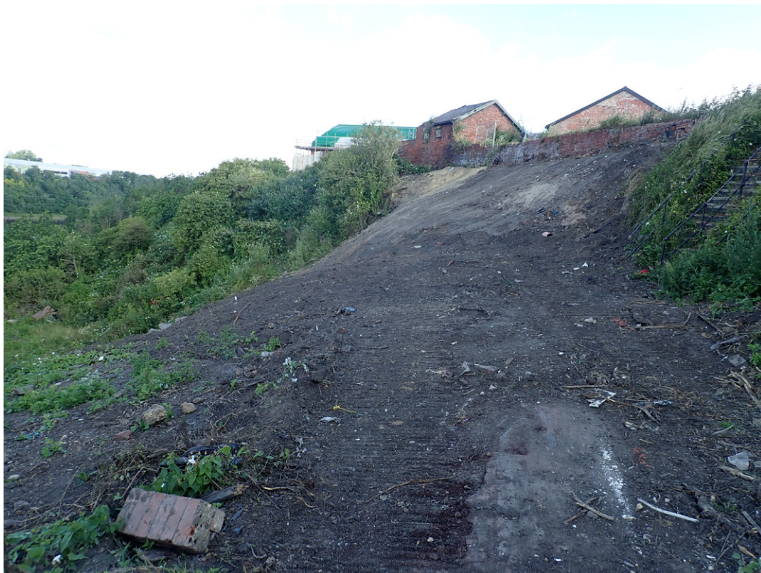
Fig. 3.32: North Abutment before excavation, facing north-west
