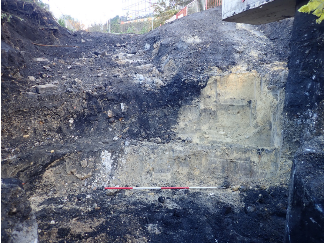
Fig. 3.41: West facing representative section in South Pier pit showing Made Grounds 402 and 403, approximately 5.5m below ground level
