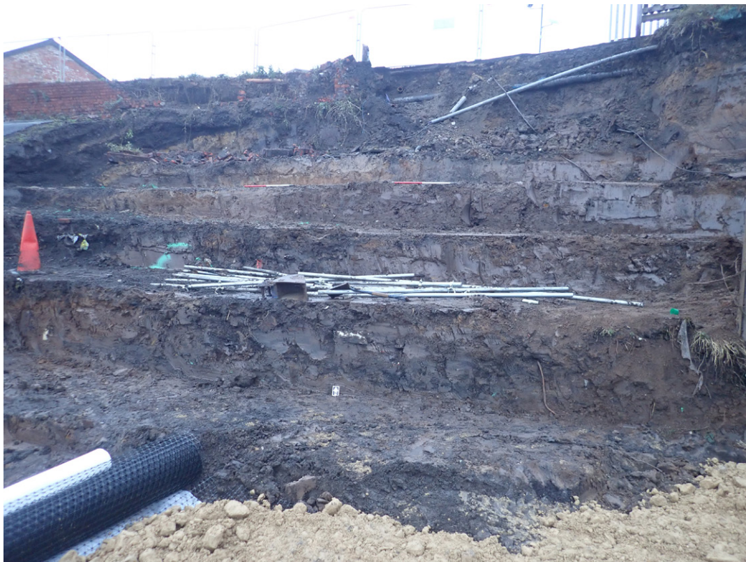
Fig. 3.34: Excavation to required depth in North Abutment, facing north
