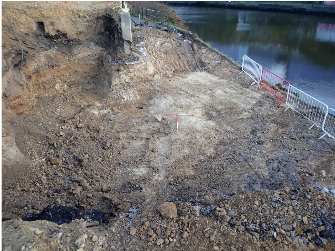
Fig. 3.24: Excavation to required depth in North Pier, facing south-east
