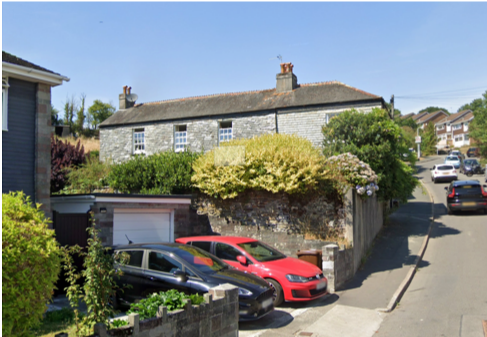
Pic 2. The south elevation, late C19 extension to right side, slate hanging, hornless 12 pane sashes to C19 main house with 4 pane sash extension
