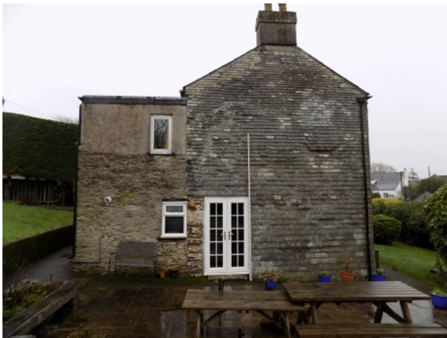
Pic 2. The south elevation, late C19 extension to right side, slate hanging, hornless 12 pane sashes to C19 main house with 4 pane sash extension
