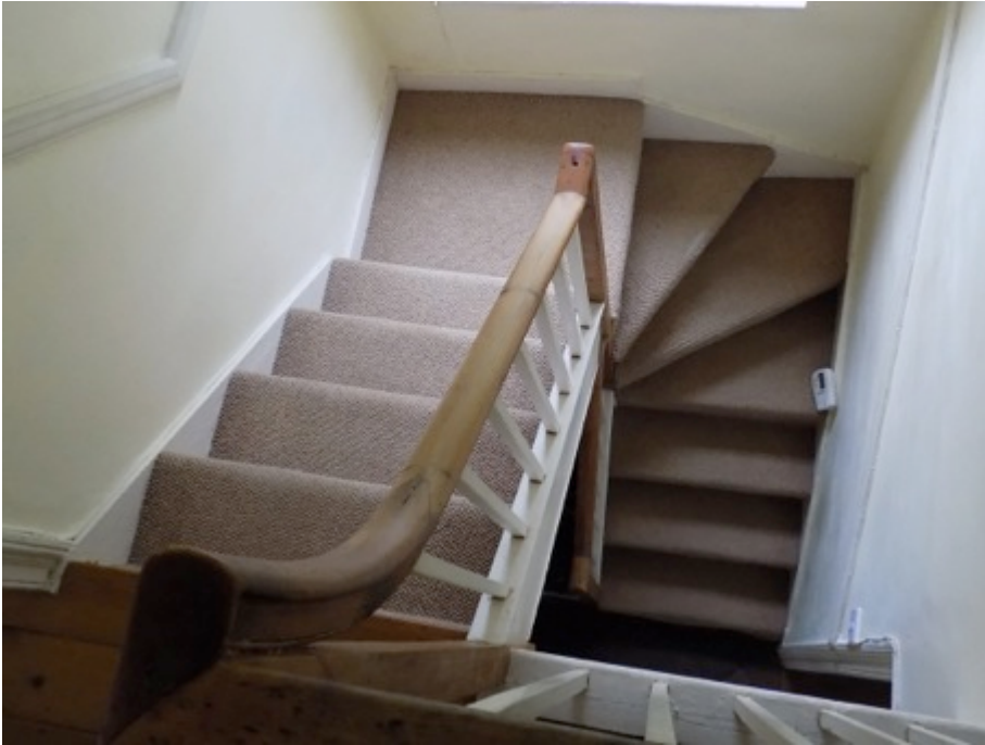
Pic 6. Existing main staircase, stick balusters and thin continuous handrail
