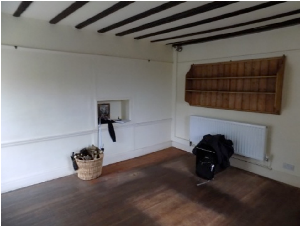
Pic 5 The evidence of door opening between dining room and rear kitchen.
