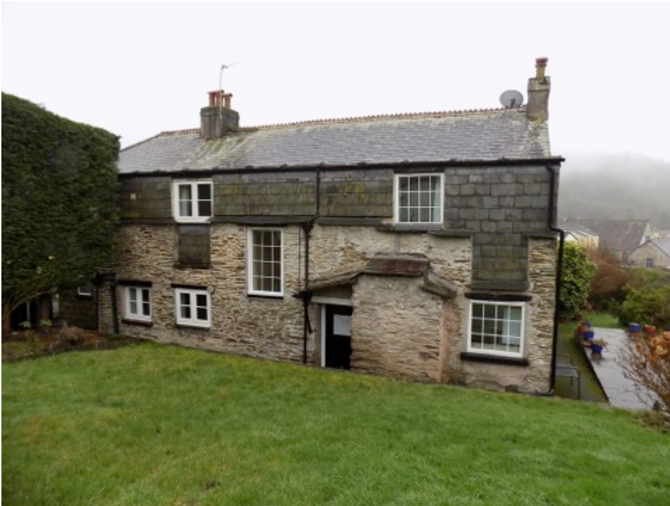
Pic 4. Extensively altered North (rear) elevation with raised slate clad extension and mix of window openings and forms.
