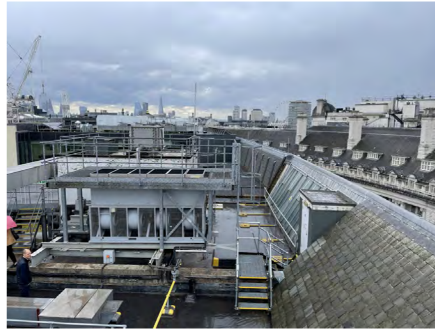
Proposed area of 7th Floor Terrace on Regent Street, looking East.
