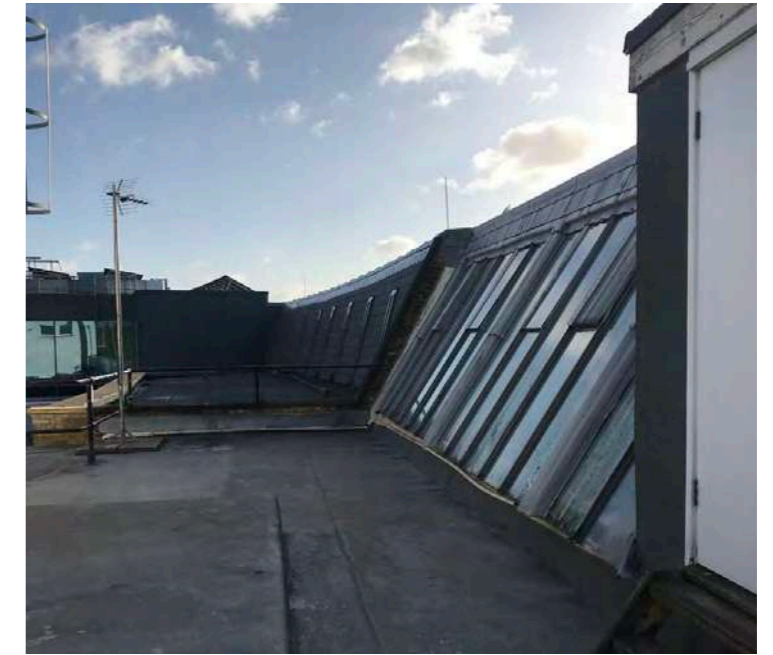
Proposed area of 7th Floor Terrace on Regent Street, looking East.
