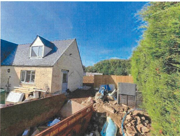
Photograph 5. The northern gable end of Rose Barn.
