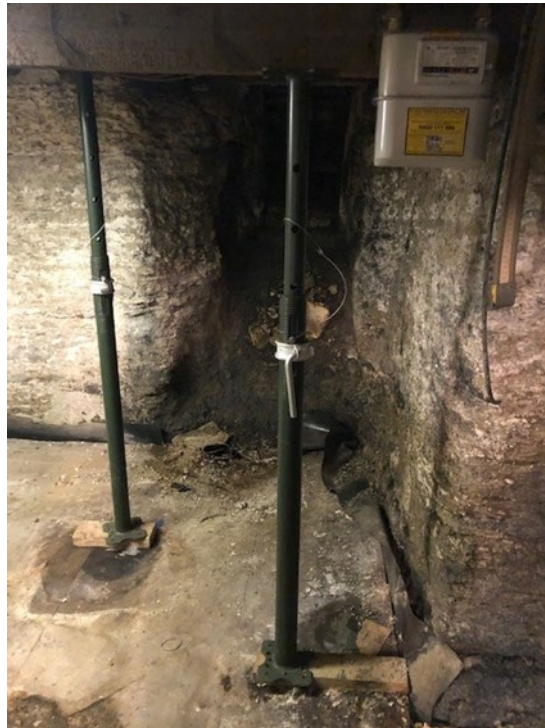
Example of acroprops currently in use in the front cellar
