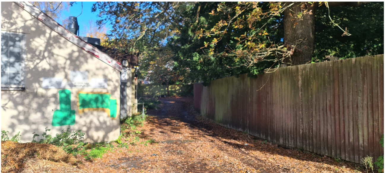
Low canopies of trees over access into middle of site. Crown lifting to canopies should be undertaken to create 4m ground clearance.
