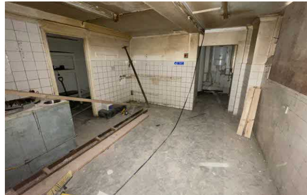
Existing modern partition to the left to be removed
