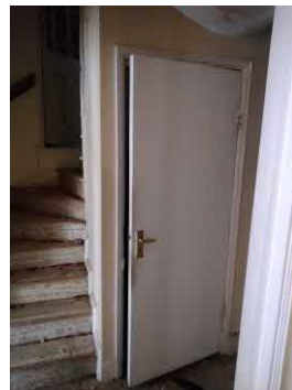
Modern door to basement stair removed
