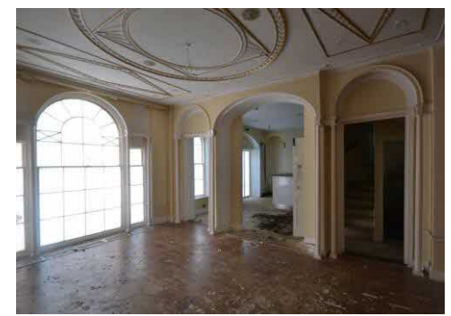
Right hand opening infilled with false door
