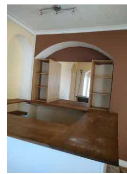
Wall to be retained
