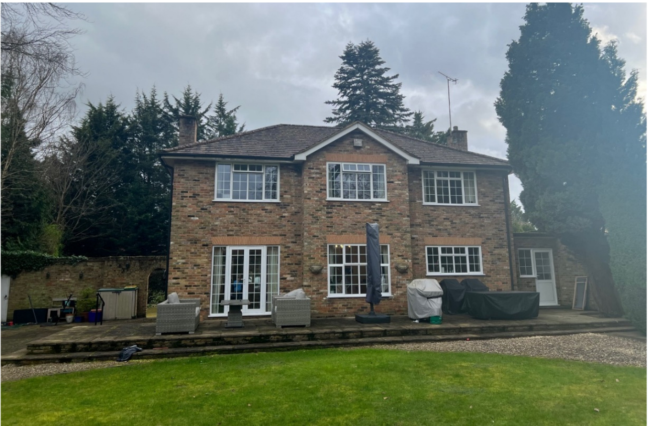
Figure 4 – View of Whiteoaks from the rear garden (North)
