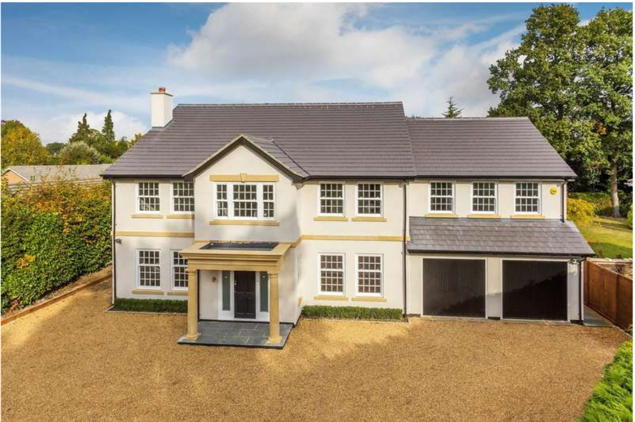
Figure 9 – View of Hentley House in Heathfield close from the front (South)
