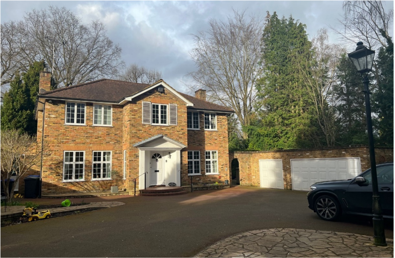
Figure 3 – View of Whiteoaks from the front (South)
