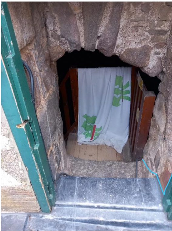
Fig. 11 Cap House doorway
