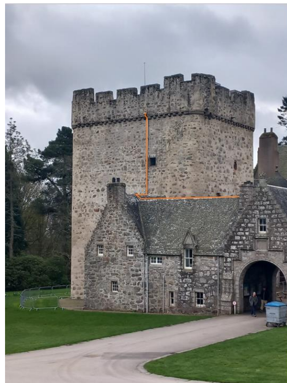
Fig.20 Cabling route from downpipe across bewhouse roof, holiday flat roof and into Tower Store above pend.
