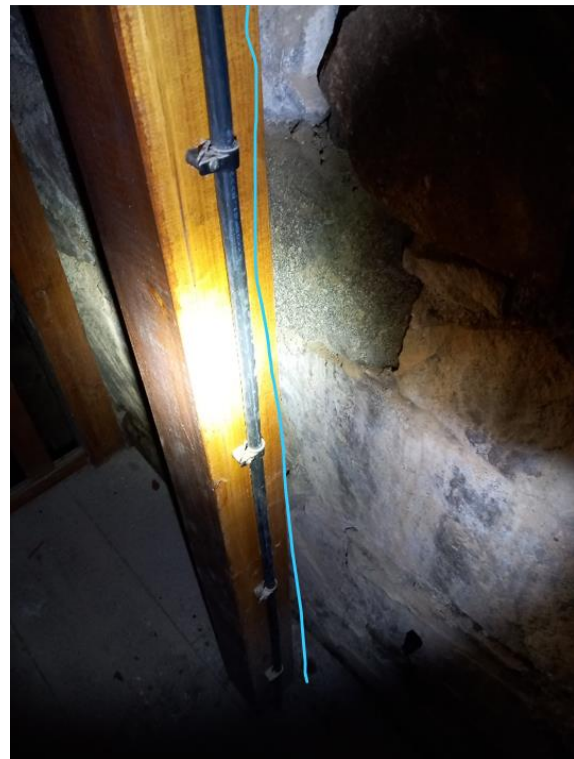
Fig. 12 Existing power cable attached to staircase
