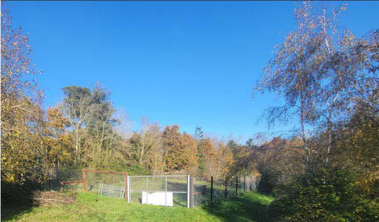
Figure 3.11 – Emergency Access Gate
