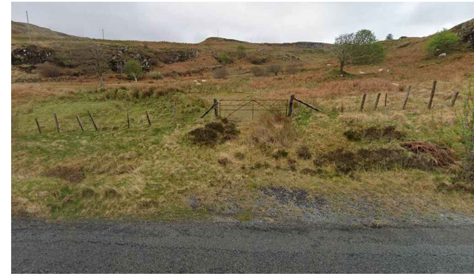
1. Existing field access to be utilised as site entrance.
