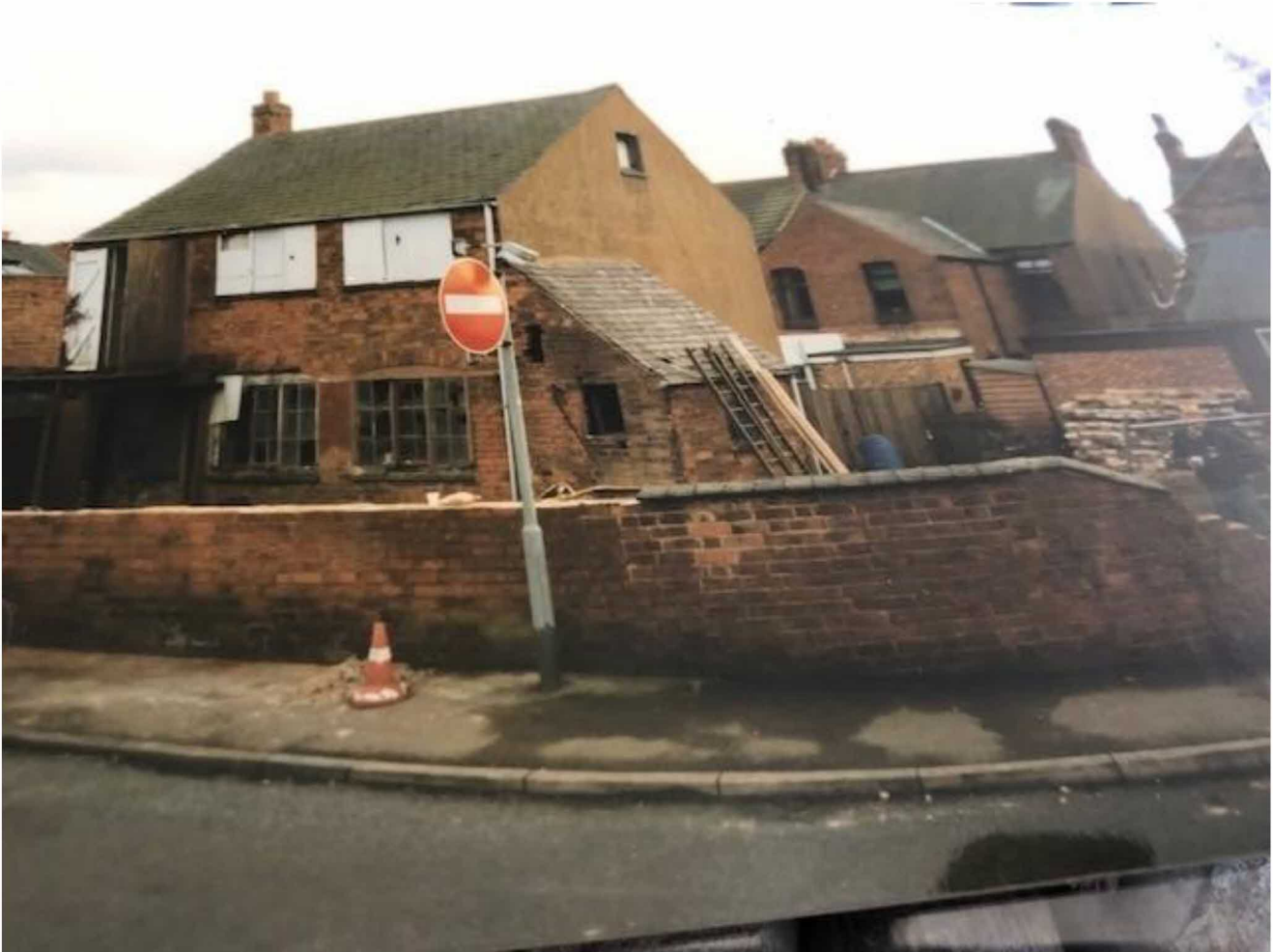
Building prior to renovation as nursery by the current applicant taken on purchase in 1996.
