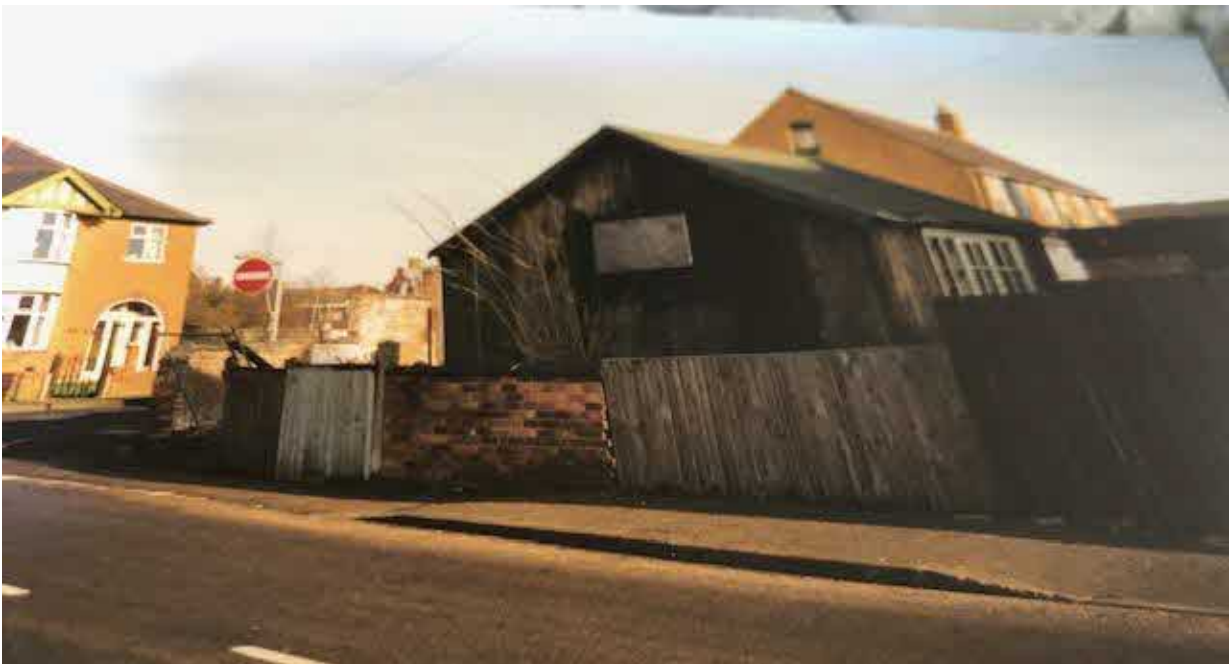
Previous single storey structure on the site
