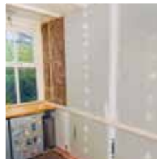
3. Plasterboard finish
