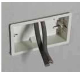
Figure 25 A plasterboard socket box
