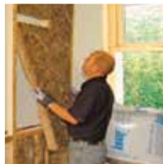
2. SWIP Batt between SWIP Studs
