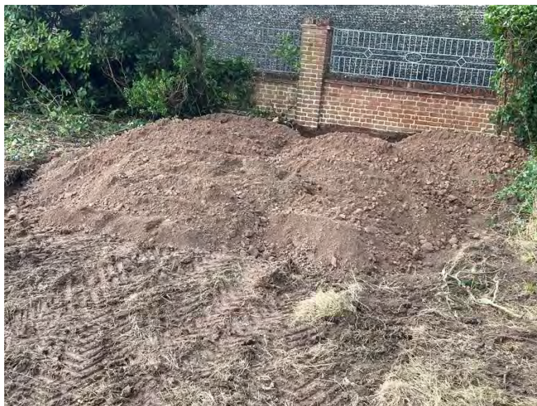
Figure 6 - Image showing sub-base aggregate.
