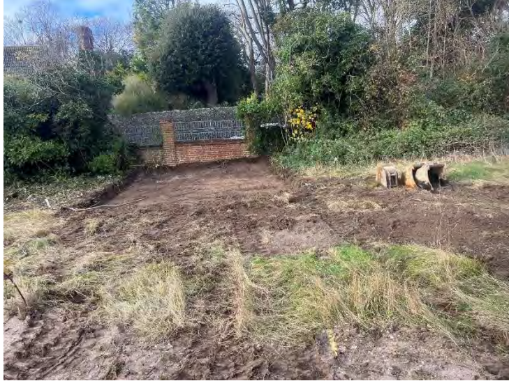
Figure 7 - Image showing ground preparation
