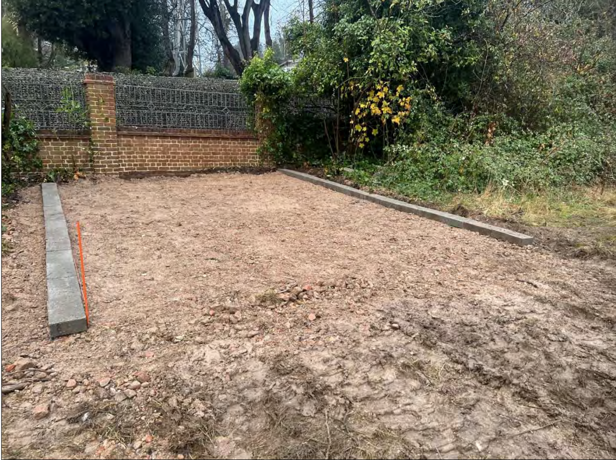
Figure 2 - Temporary kerbs and sub-base material
