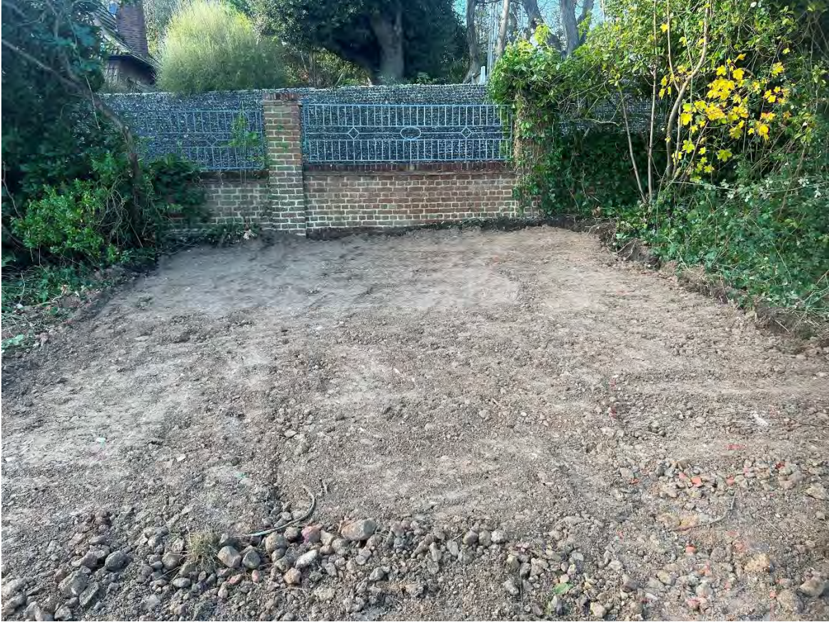
Figure 5 - Image showing the stage the sub-base was constructed
