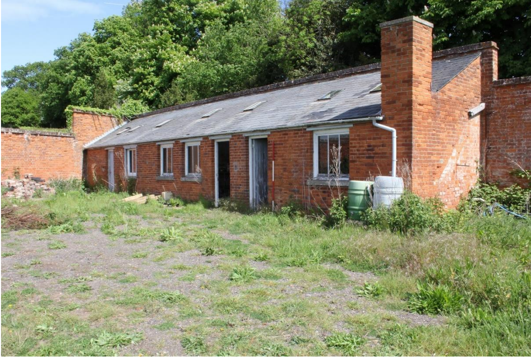
Plate 17 External ancillary building, looking north. Scale 2m
