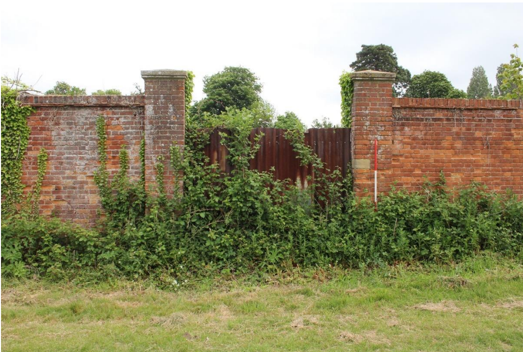
Plate 2 External southern double gated entrance, looking north-east. Scale 2m
