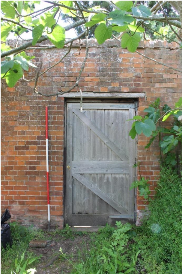
Plate 11 Internal northern pedestrian gated access looking north-east. Scale 2m
