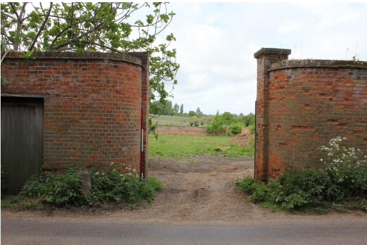
Plate 6 External northern double gated access, looking south-west. Scale 2m
