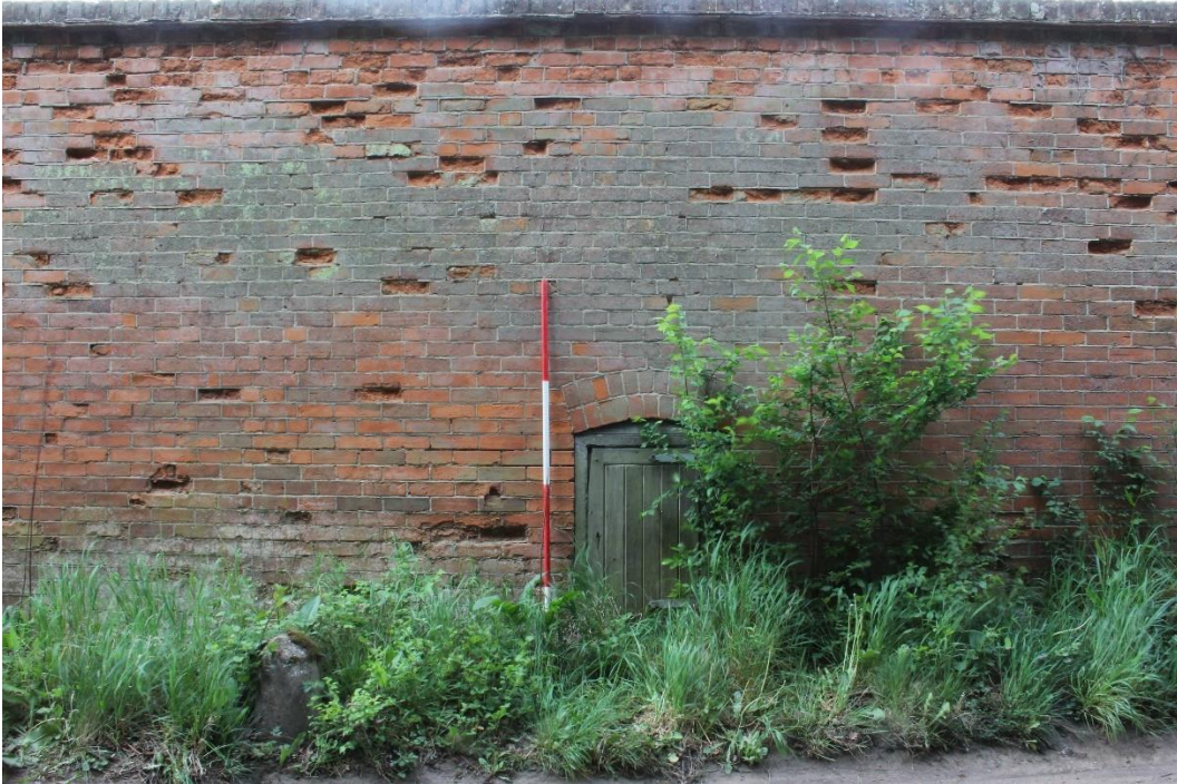
Plate 7 External northeast wall showing coal shoot door, looking south-west. Scale 2m
