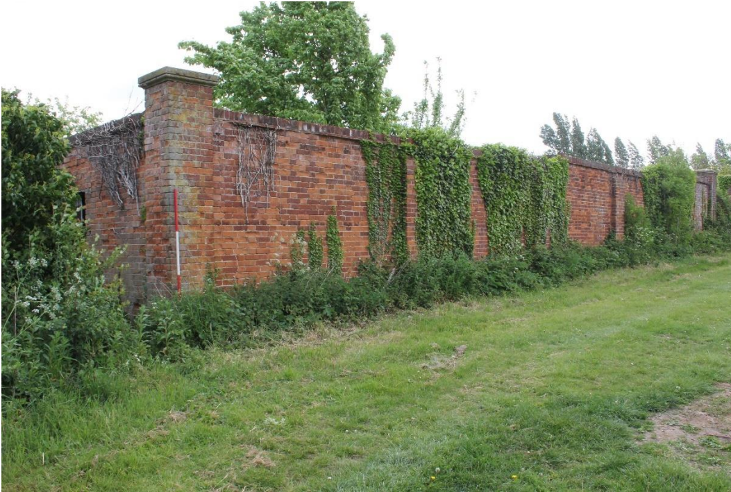
Plate 1 External wall at south-west corner, looking north-east. Scale 2m
