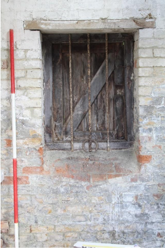
Plate 23 Internal barred coal shoot door within room 4, looking north-east. Scale 2m
