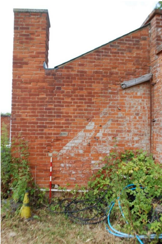
Plate 24 South-east facing wall of ancillary building showing paint from former structure, looking north-west scale 1m
