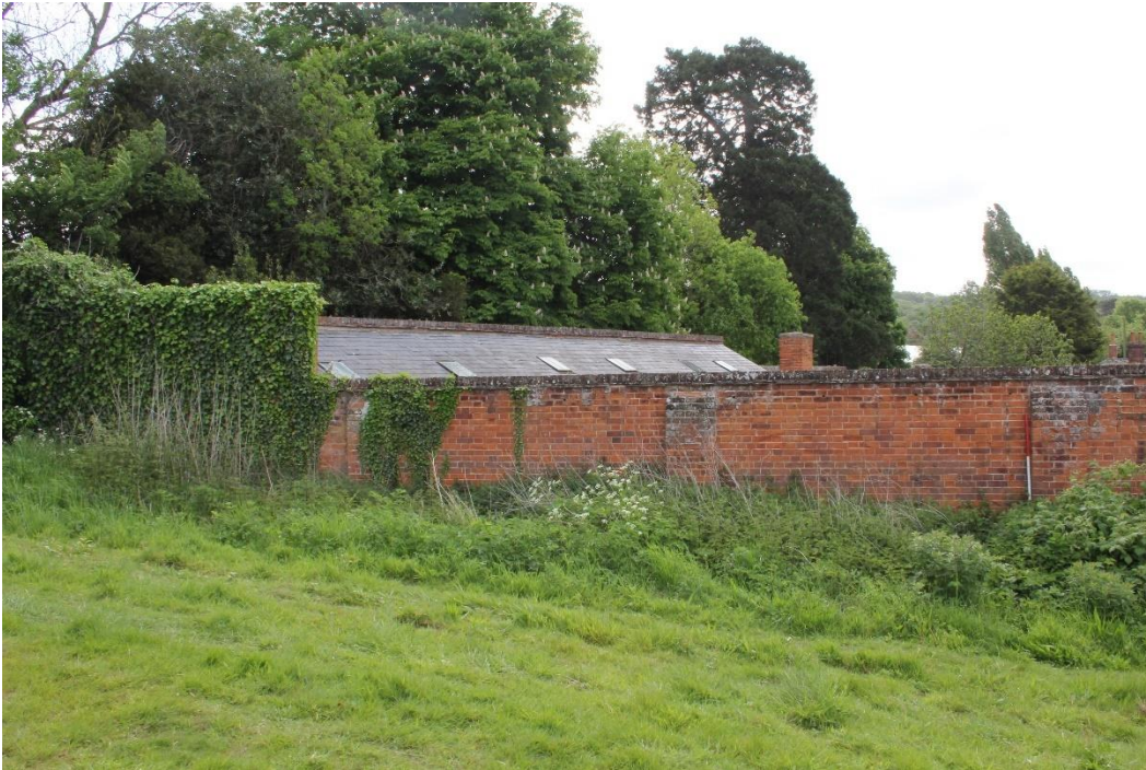
Plate 9 External north-west wall with ancillary building beyond, looking south-east. Scale 2m
