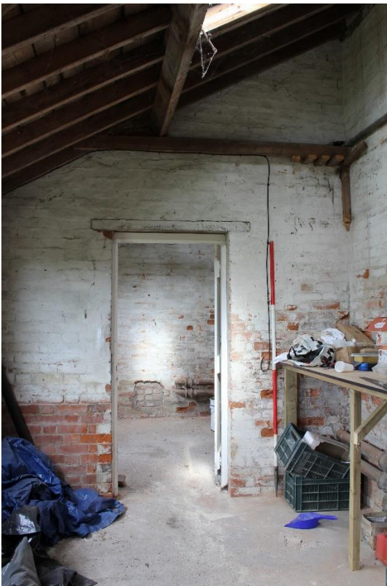
Plate 22 Internal room 3 and doorway to room 2, looking north-west. Scale 2m
