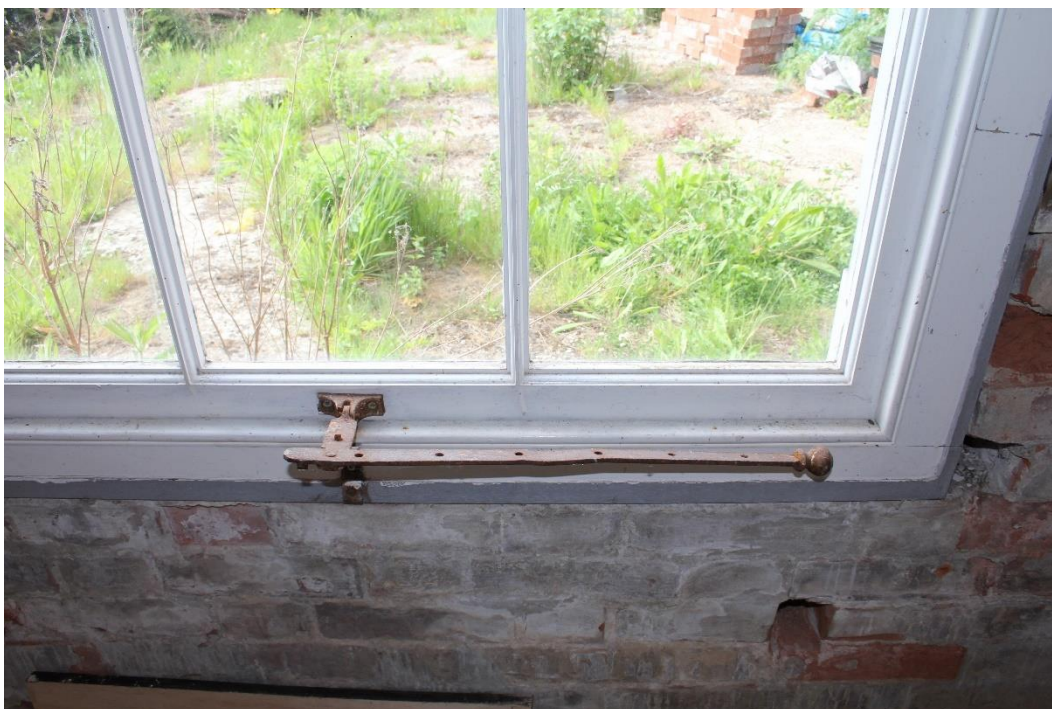
Plate 20 Internal casement window showing a possibly original latch, looking south-west
