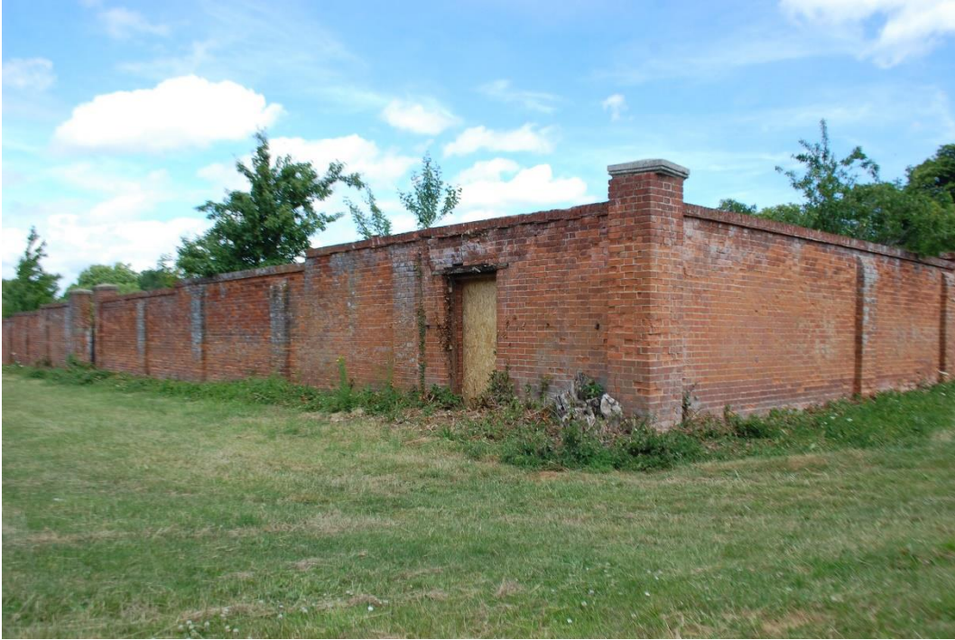
Plate 3 External wall at south-east corner, looking north.
