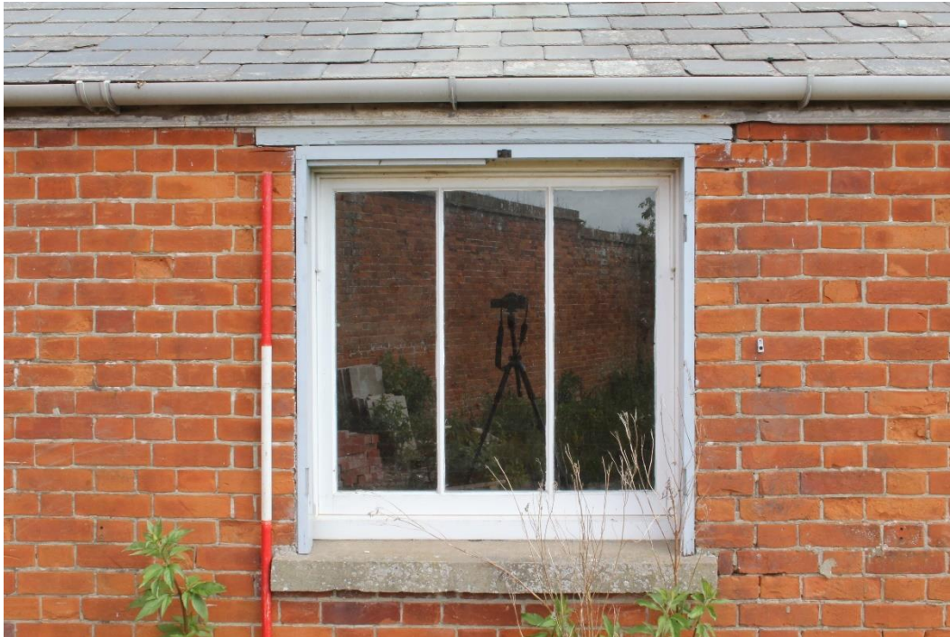
Plate 19 External casement window, looking north-east. Scale 2m (showing the upper 1m)
