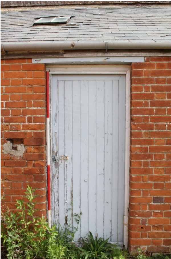
Plate 18 External door into room 1, looking north-east. Scale 2m
