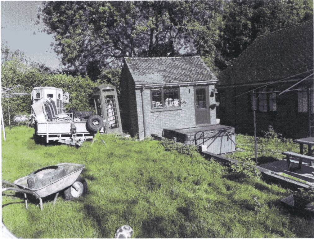
rear roof of bungalow and detached outbuilding to the rear
