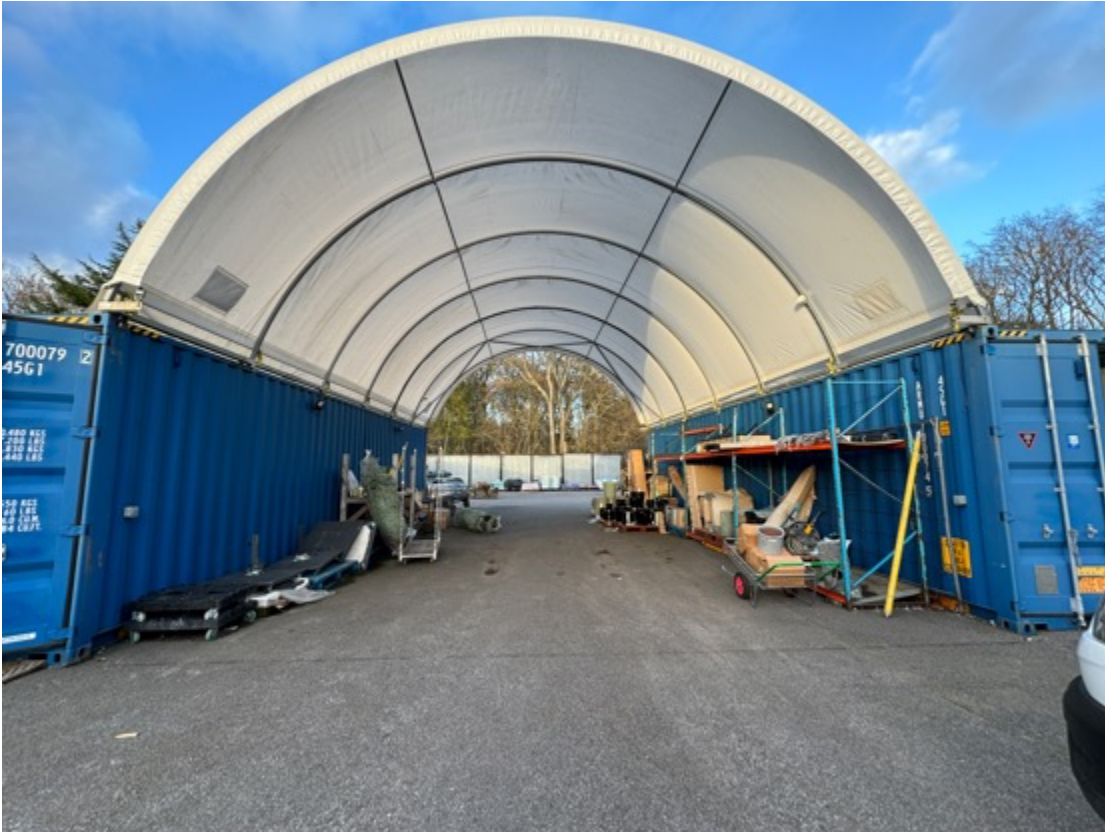
Photograph 1: Illustrating the metal storage containers and the adjoining fabric canopy
