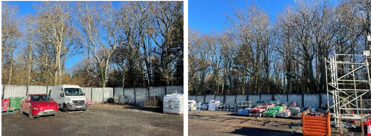
Photos 1 & 2: Trees and woodland surrounding proposed site, existing hard surfacing to be lifted using hand tools only – AMS provided.
