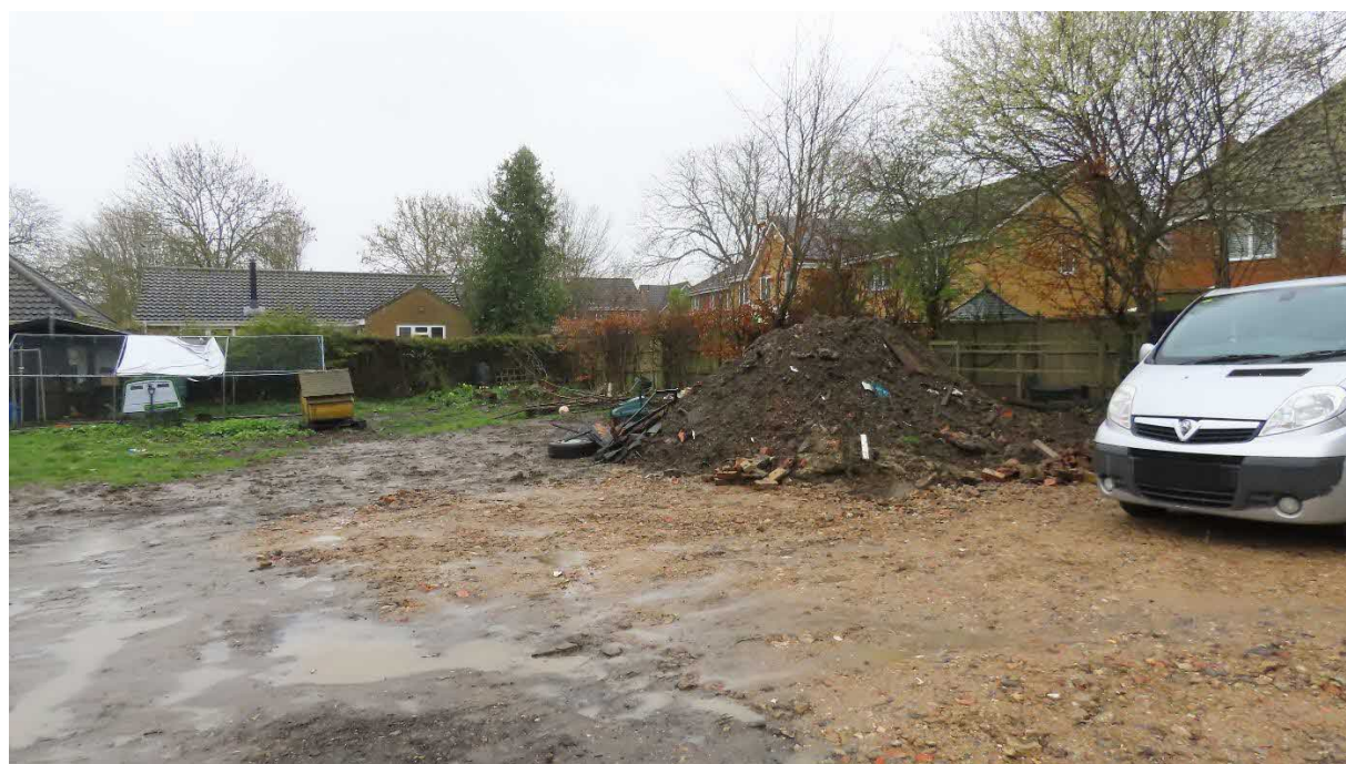
Photograph 2. General view of site including the rubble and spoil pile
