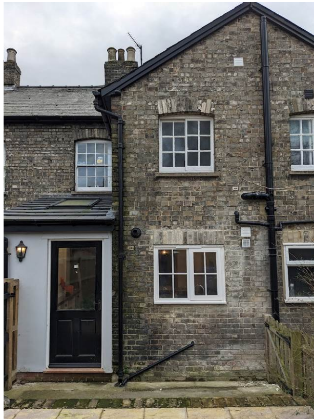
'As built' extension
