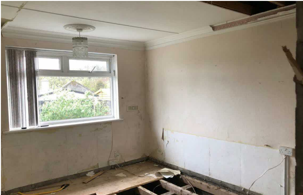
Figure 7: Interior of the building at ground level showing partial ceiling.
