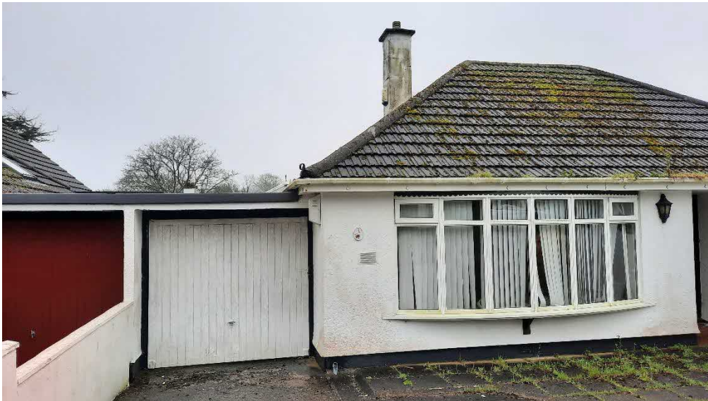
Figure 3: North-east elevation of the building showing adjoining flat-roofed garage.
