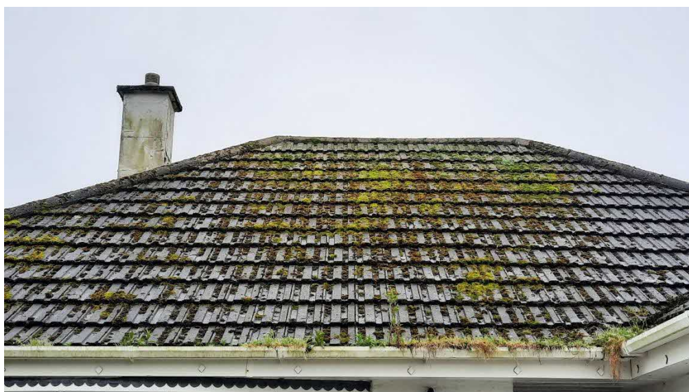
Figure 5: North-east facing roof slope showing interlocking tiles with some moss coverage.
