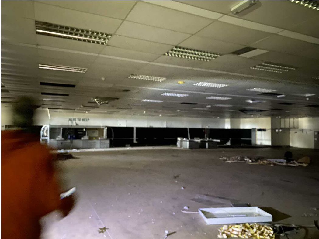
Upper ground floor interior photo 1
