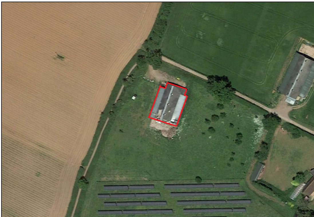
Figure 1. Location of the building. GoogleEarth June 2022.
