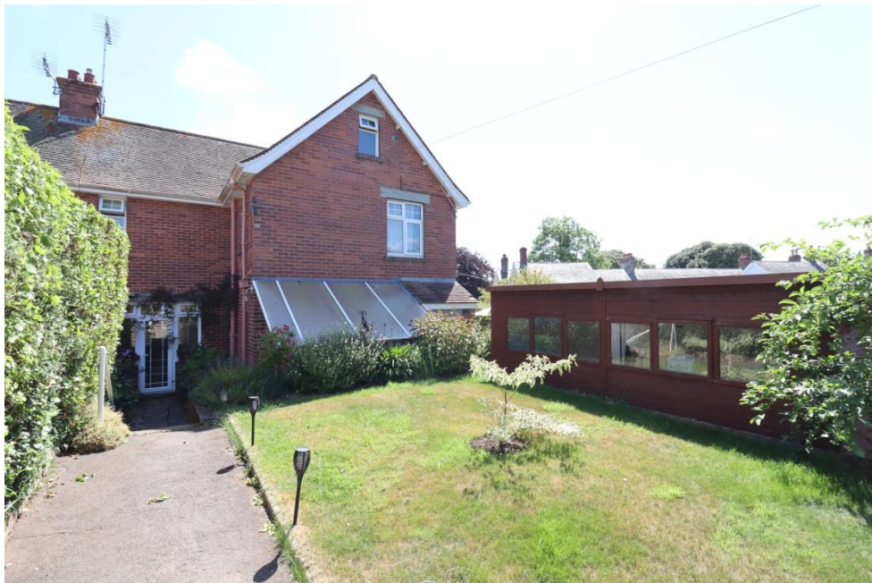
Photograph 4: Existing west elevation viewed when entering from pedestrian gate
