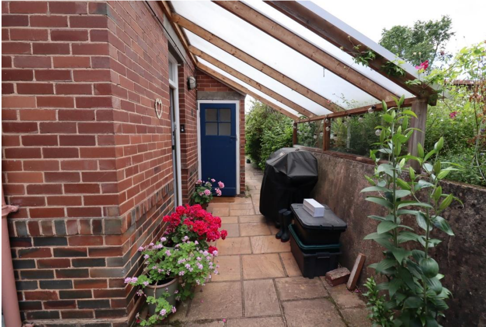
Photograph 5: Existing lean-to porch structure and externally accessed W/C
