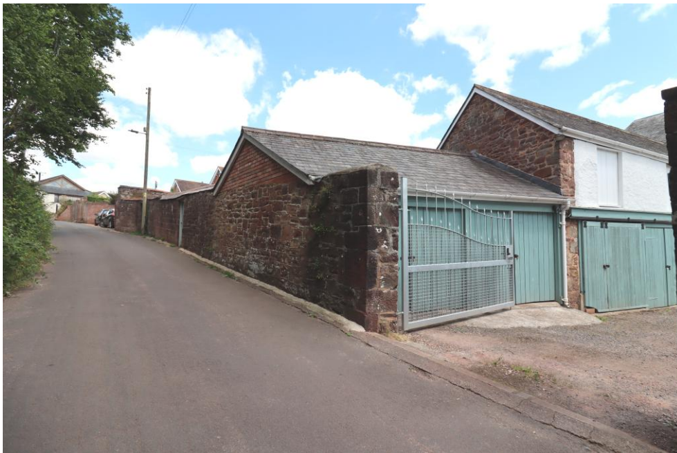
Photograph 10: Characteristic brick and stone walling continuing to neighbouring Taw Vale Terrace to the south of Yeo Vale
