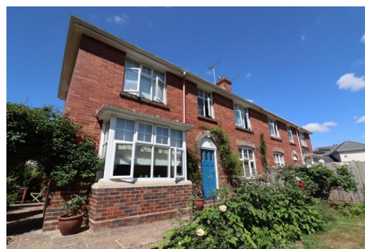
Photograph 2: East facing arts and crafts facade
