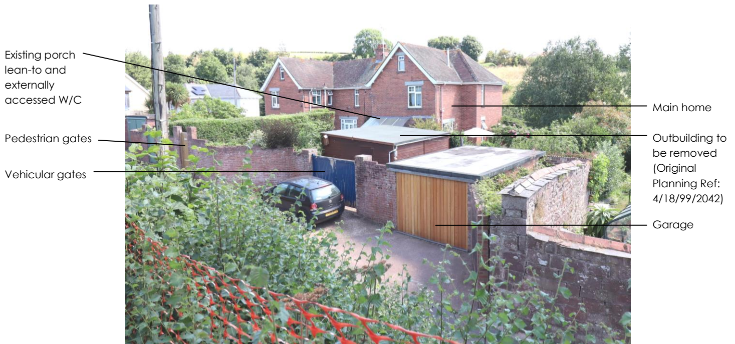
Photograph 1: Overview of west side of Yeo Vale
