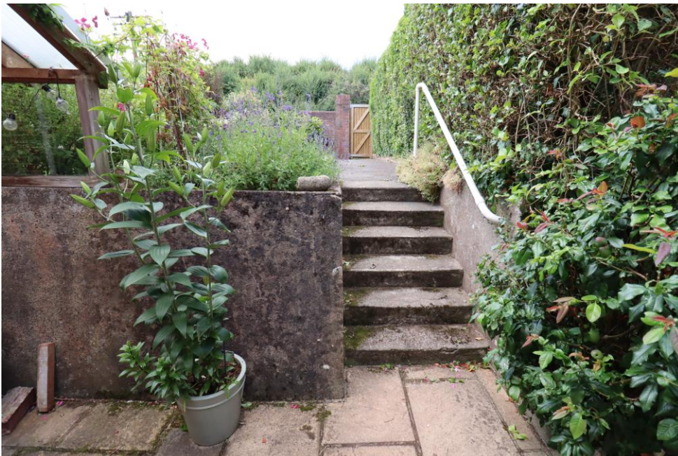
Photograph 8: Existing steps along pedestrian access path
