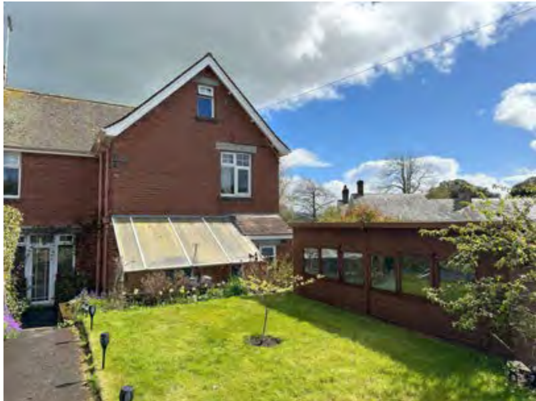
P.1 Western elevation and current lean-to.
