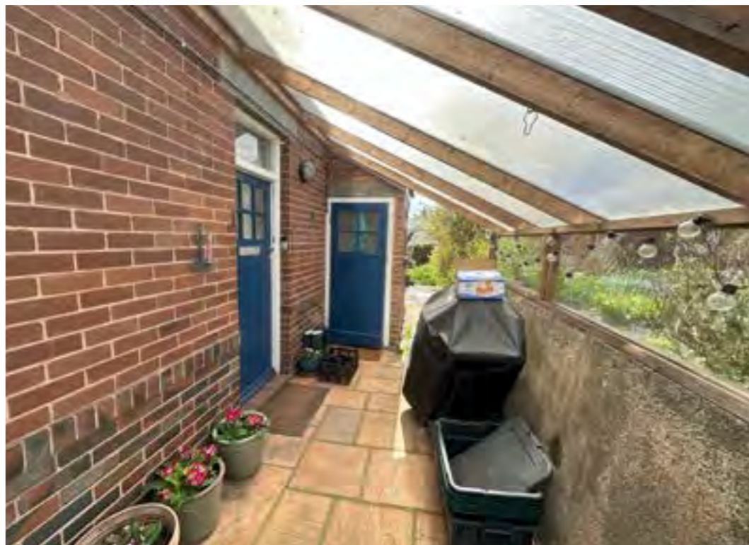
P.3 View South toward boundary wall of Taw Vale Terrace
