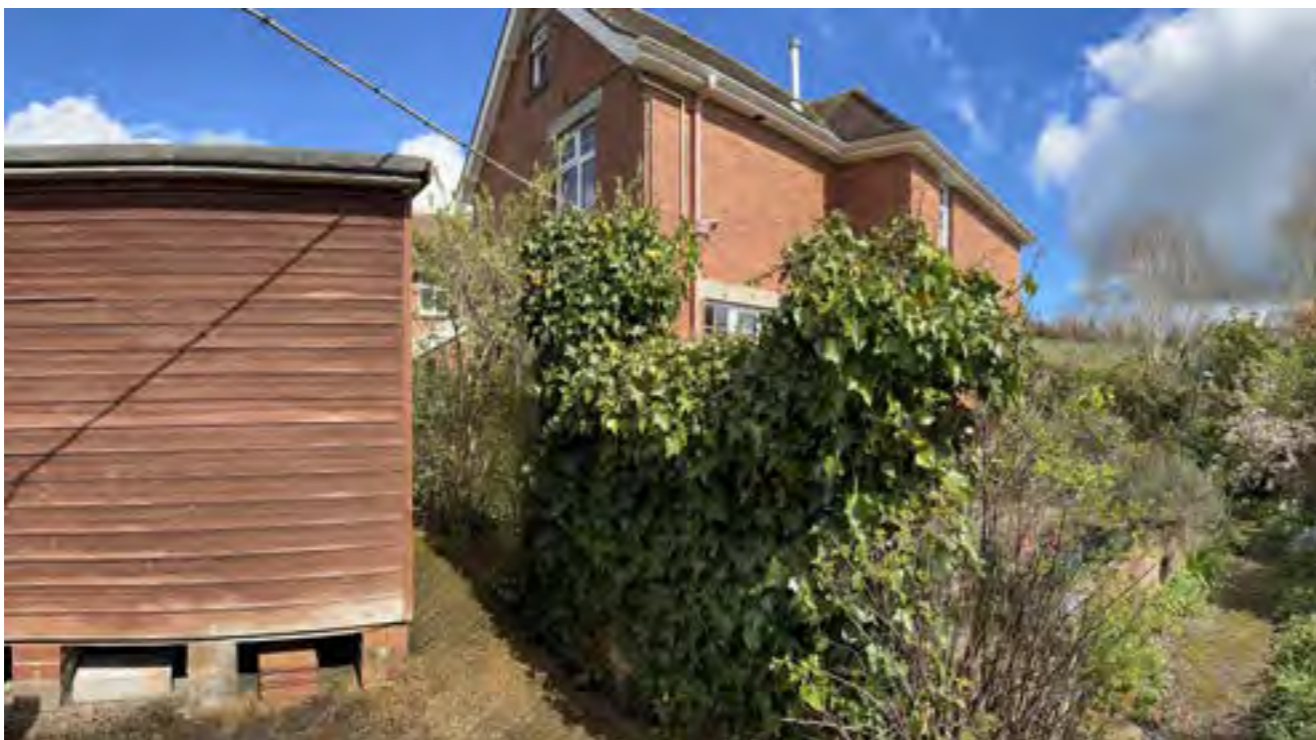
P.7 View north from boundary wall toward porch area.
