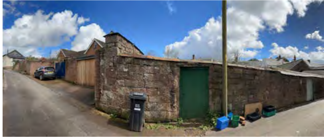
P.9 Boundary wall onto Four Mills Lane of Taw Terrace building(s).
