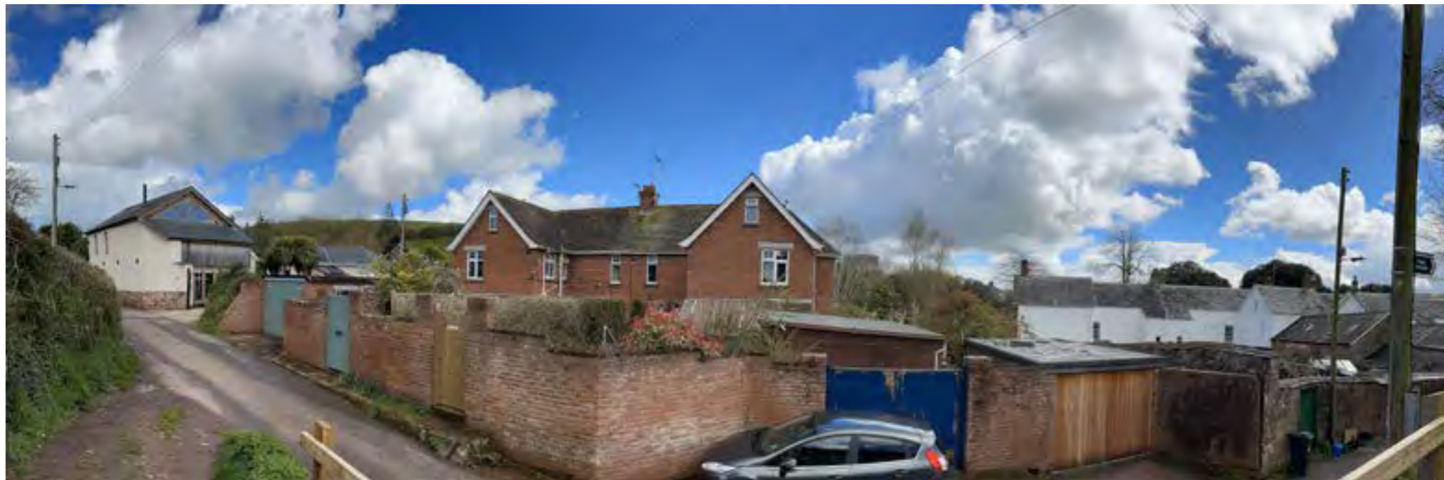
P.10 General Panarama east over Yeo Vale and Taw Terrace(s)
