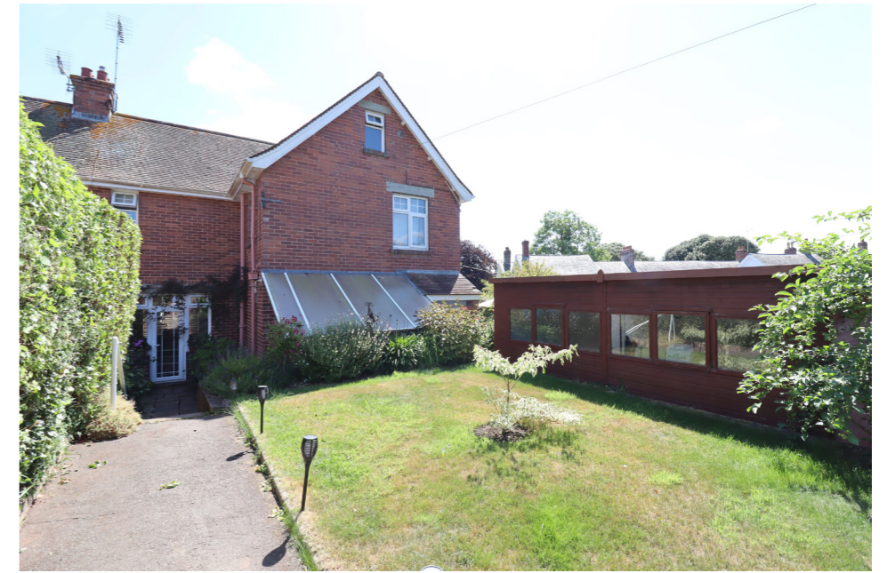
Photo 3: Existing west elevation viewed when entering from pedestrian gate
