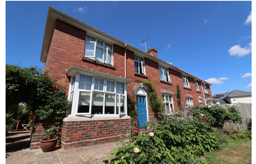
Photo 6: View of existing east elevation which was originally the front elevation and is to be unchanged by the proposals
