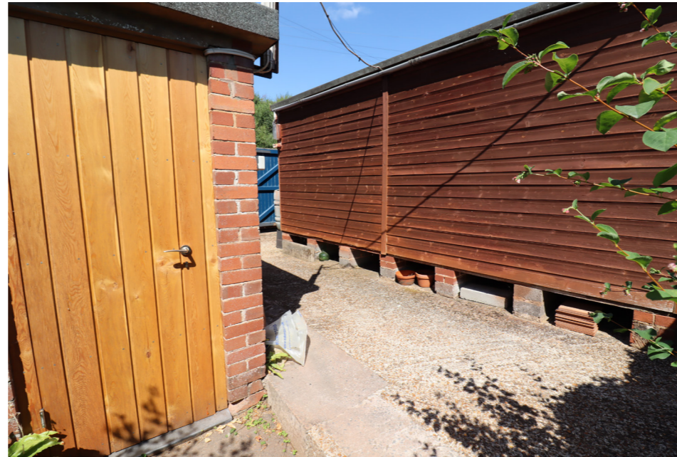
Photo 5: View of existing timber outbuilding to be demolished
