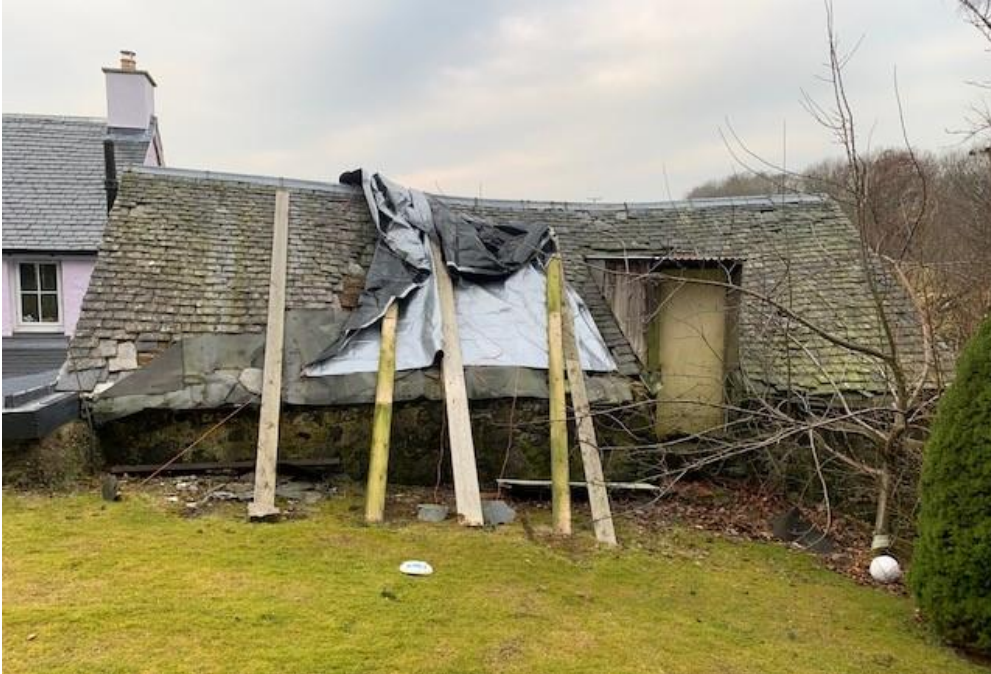
Photo 3. The northern side of the garage.
