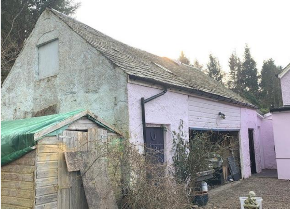
Photo 1. The south and west side of the garage.
