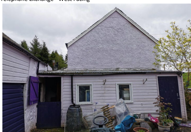
North Gable – Cottage of Clunie.
