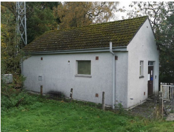
Telephone exchange Building – North Facing
