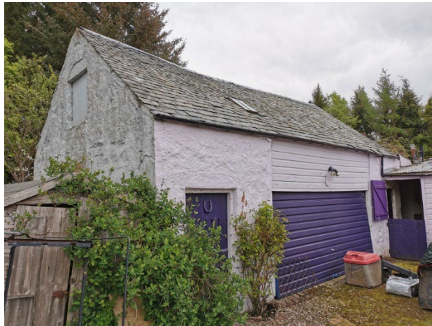
Existing Garage Outbuilding as viewed from Northwest
