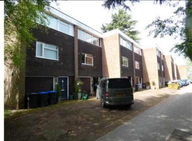
Photograph 2. The east elevation of the building (from north-west corner)
