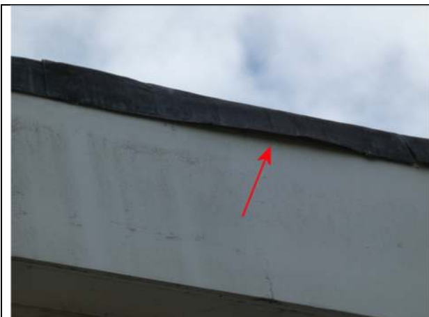
Photograph 29. Opening under the roof edge trim on the east elevation of Nos 7 and 8
