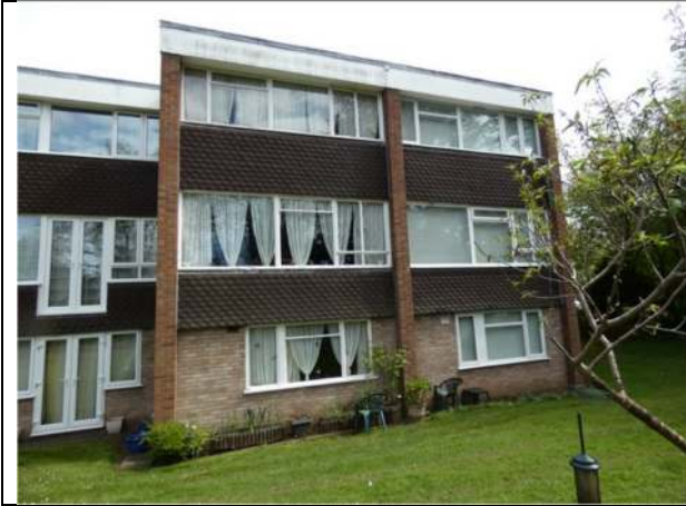
Photograph 7. The west elevation of Nos 1 and 2
