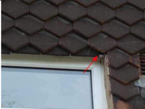
Photograph 49. Opening under hanging tiles at the corner of a window on the east elevation of Nos 13 and 14
