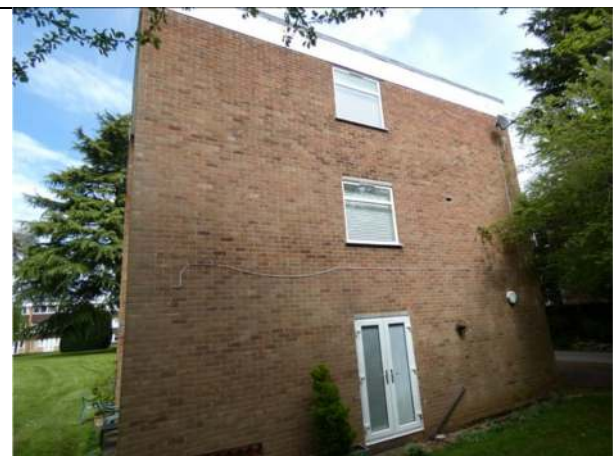
Photograph 6. The south elevation of Nos 1 and 2
