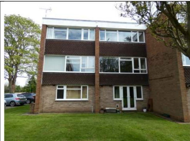
Photograph 45. The west elevation of Nos 13 and 14
