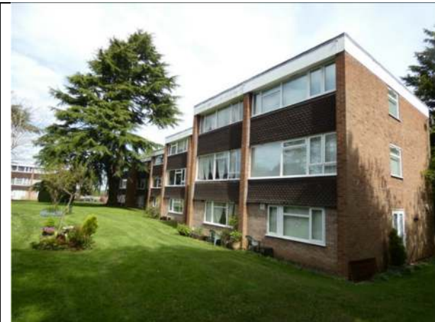
Photograph 3. The north and west elevations of the building (from north-east corner)
