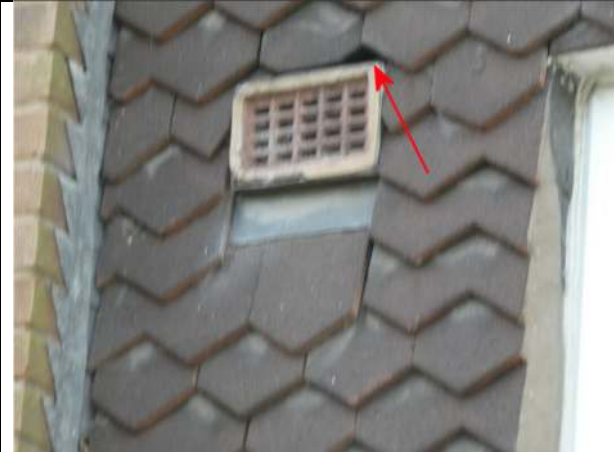
Photograph 31. Opening above the vent on the east elevation of Nos 7 and 8
