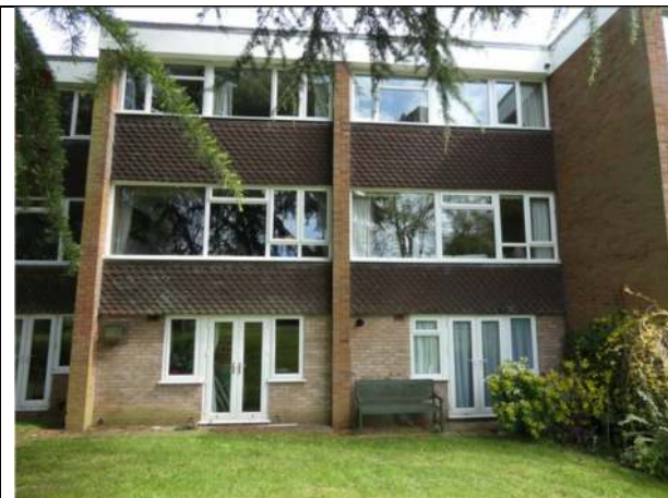
Photograph 21. The west elevation of Nos 5 and 6
