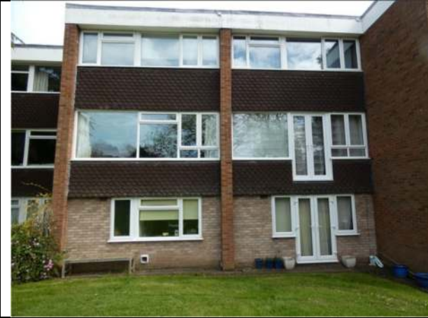
Photograph 13. The west elevation of Nos 3 and 4
