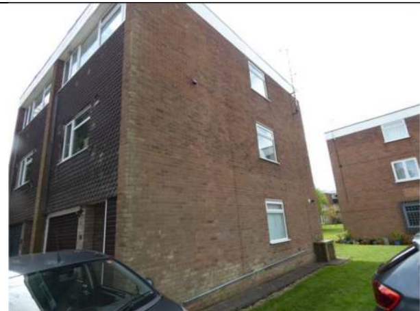
Photograph 46. The north elevation of Nos 13 and 14
