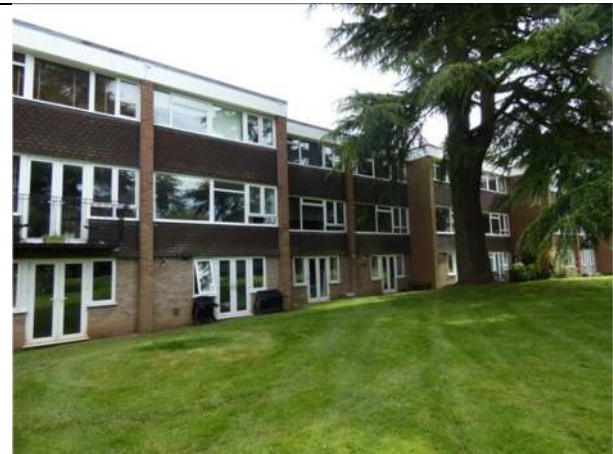
Photograph 4. The east elevation of the building (from southern end)
