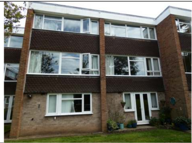
Photograph 40. The west elevation of Nos 11 and 12
