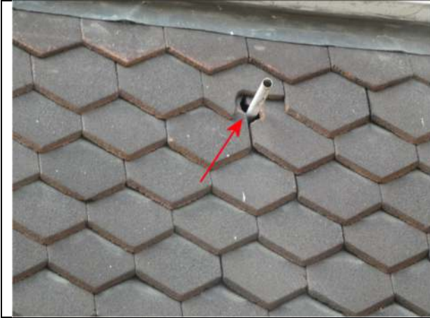
Photograph 25. Opening in the hanging tiles on the east elevation of Nos 5 and 6
