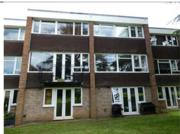
Photograph 36. The west elevation of Nos 9 and 10
