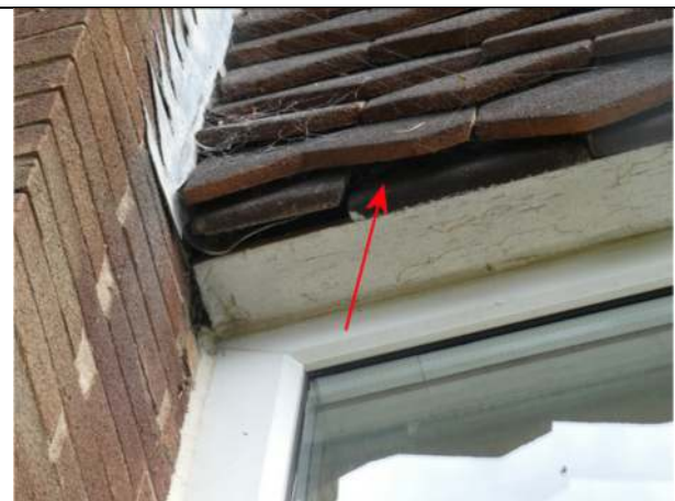
Photograph 42. Opening under hanging tiles on the west elevation of Nos 11 and 12
