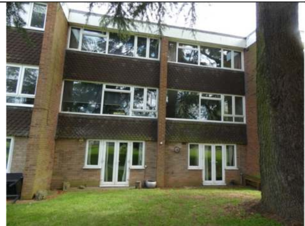
Photograph 28. The west elevation of Nos 7 and 8
