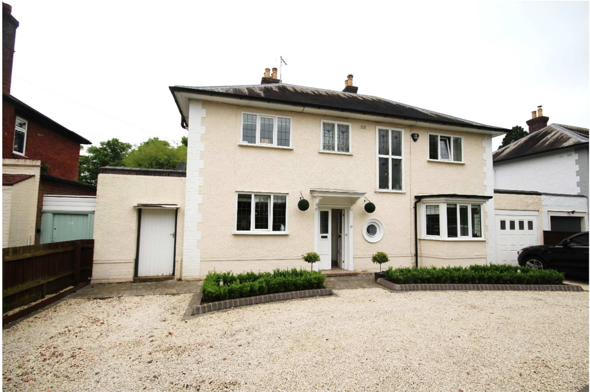
View 2 – View from drive
