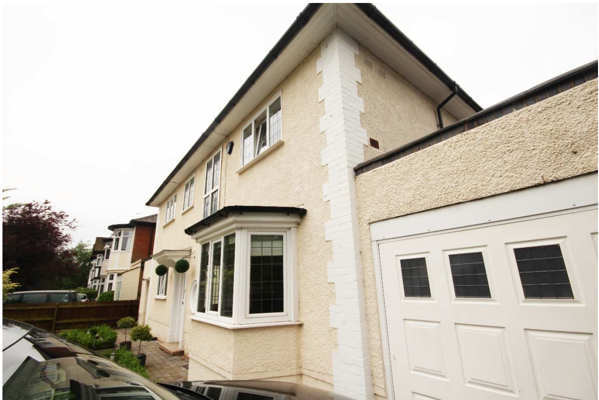
View 3 – Detail of existing uPVC windows to front elevation
