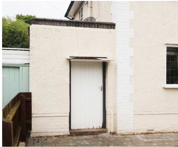
Existing utility access door to front side extension
